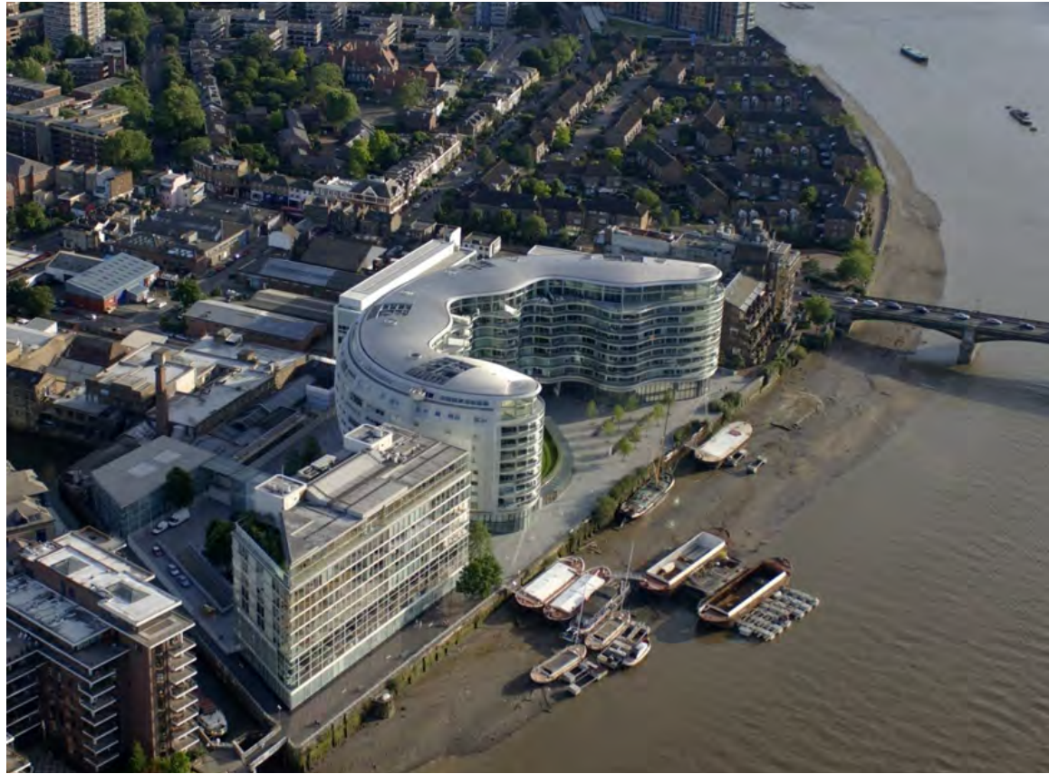
18. Foster &amp; Partners' Riverside and Albion Riverside around 2003
