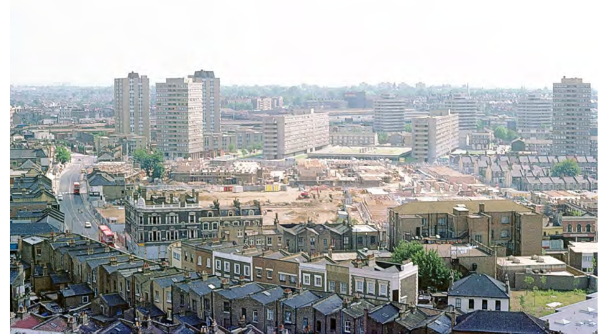
17. Public housing transforms north Battersea: looking south from near the York Road–Falcon Road junction, 1977, towards (left to right) the Livingstone, York Road Stage I and Winstanley Estates, with the Kambala Estate under construction in the middle ground
