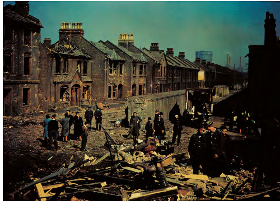
15. Bomb damage at the south end of Tennyson Street looking north, 1943
