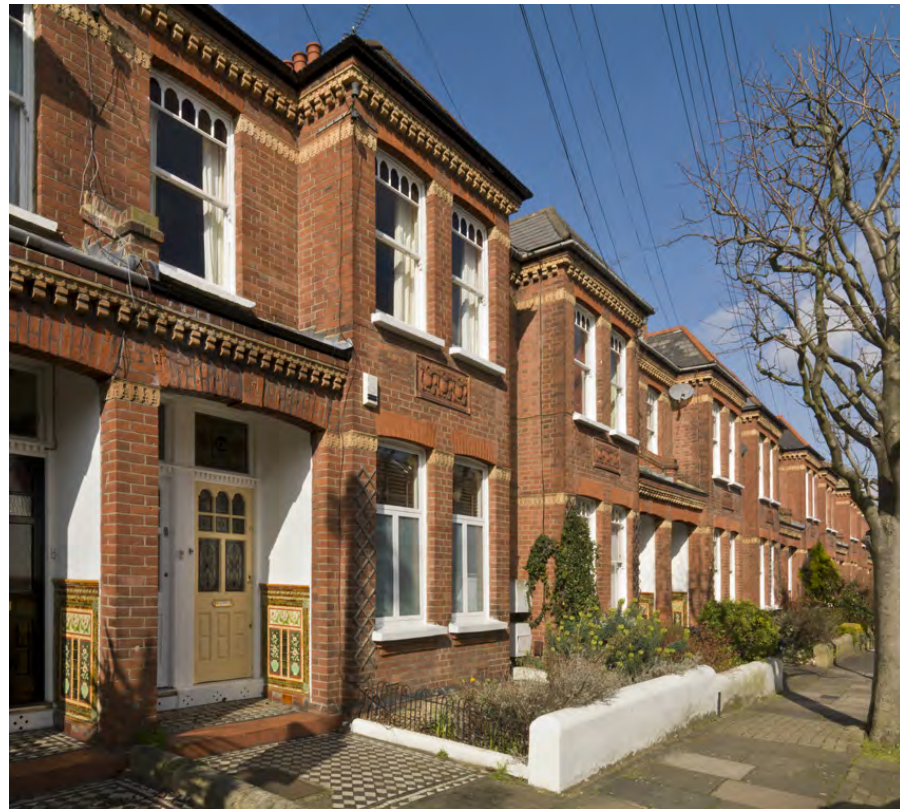
11. Cottage flats at 220–226 Boundaries Road in 2013
