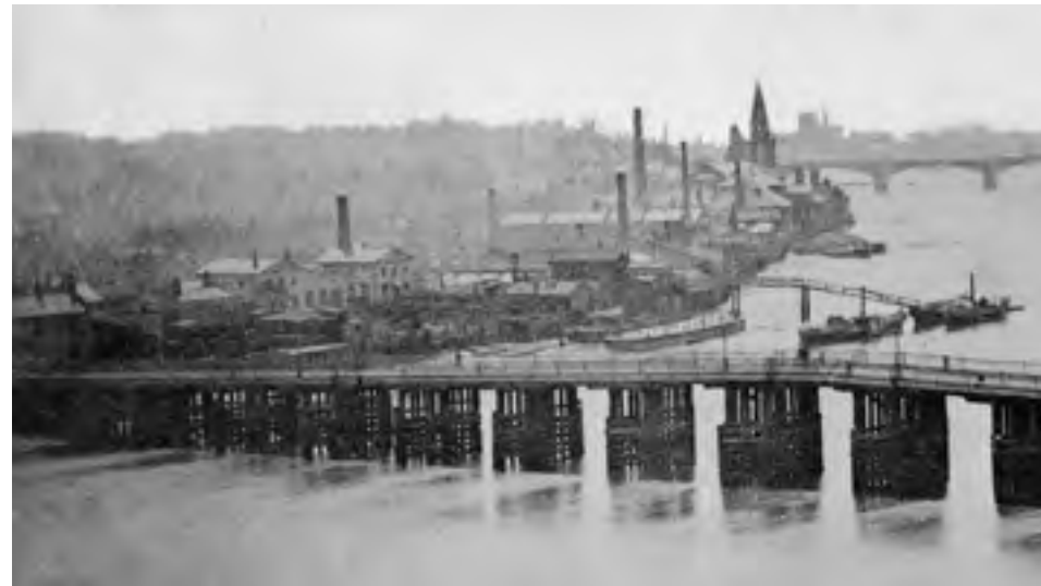
385. Thames foreshore west of Battersea Bridge, c.1870, with former Brunel sawmills left of centre, when in use by the Thames Steamboat Company. Demolished
