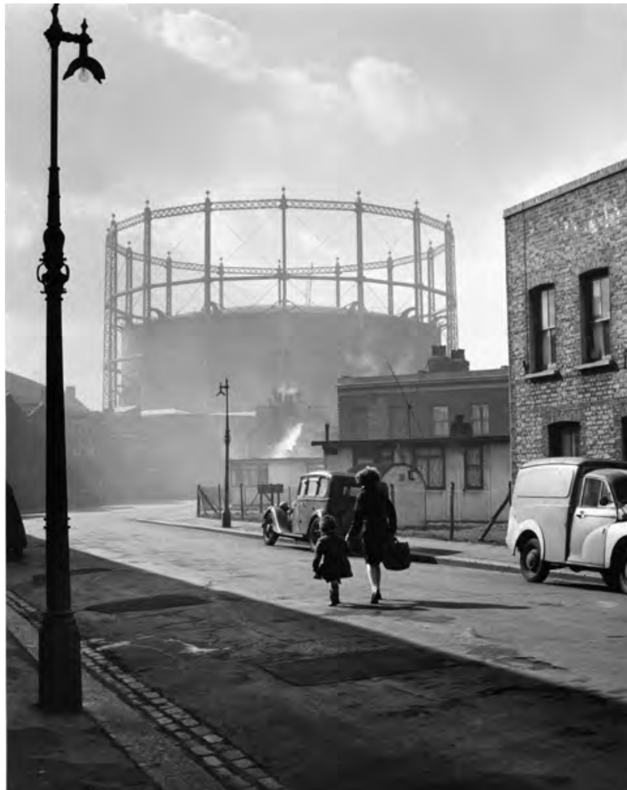
364. Nine Elms Gasworks, No. 2 gasholder of 1891–2, seen from the east (possibly Belfour Street) in 1958. Demolished
