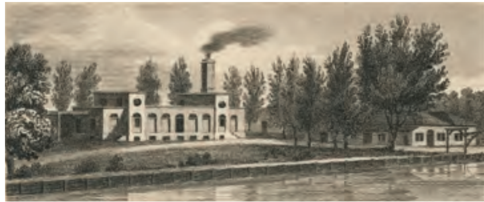
383. Marc Brunel's sawmills of 1807, view before their partial destruction by fire in 1814
