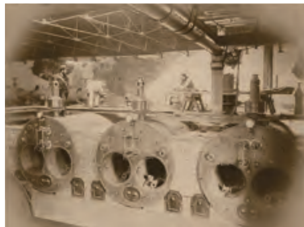
379. Lancashire boilers being installed at the Southwark & Vauxhall Waterworks, probably in 1884
