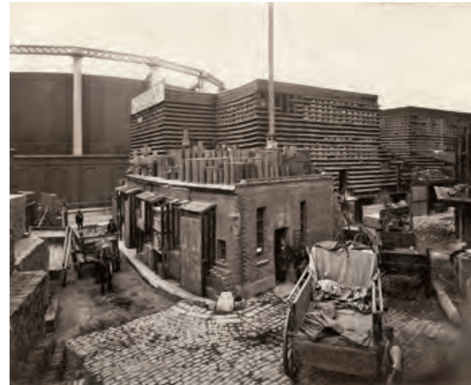
371. Laver's Wharf, Nine Elms, in 1906, looking south towards Nine Elms Lane, with gasworks (Gasholder No. 1) in the background. The tall wooden sheds, used for drying whiting at the end of its manufacturing process, were probably of eighteenth-century origin. Demolished
