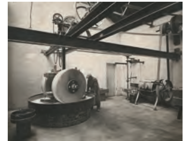
395. Mill room at Whiffen & Sons, c.1915. Demolished
