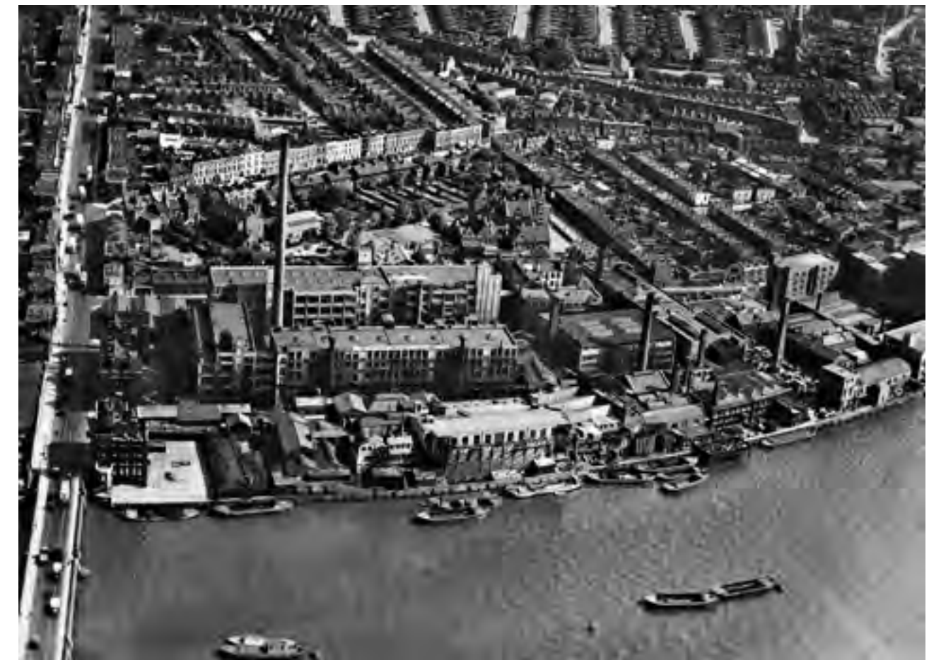
386. Morgan Crucible works from the air in 1937. The former Brunel sawmills are in front of the U-shaped factory buildings with tall chimney. Demolished
