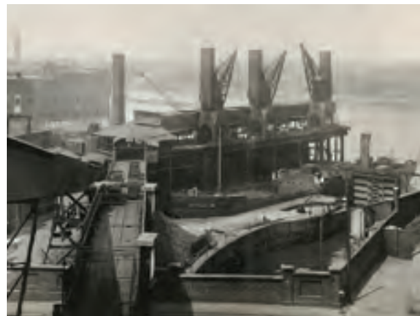
372. Nine Elms Gasworks, SS Afterglow unloading at a riverside coal wharf, c.1925. Coal conveyor over Nine Elms Lane in the foreground. Demolished
