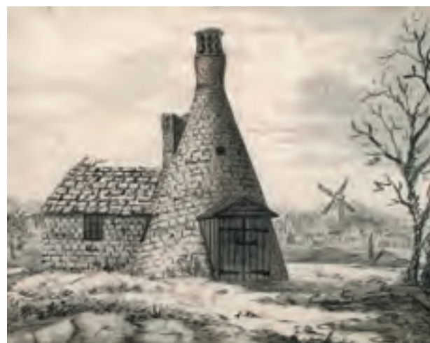
366. Early vitriol furnace in Battersea Fields, 1797, looking north towards river
