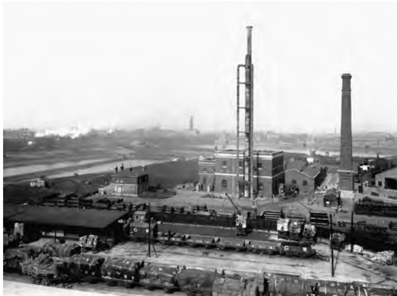
378. Southwark & Vauxhall Waterworks from the south in 1914, showing (from right to left) chimney, engine-house with standpipes in front, caretaker's cottage and reservoirs. In the foreground is part of the South Lambeth Goods Station. All demolished
