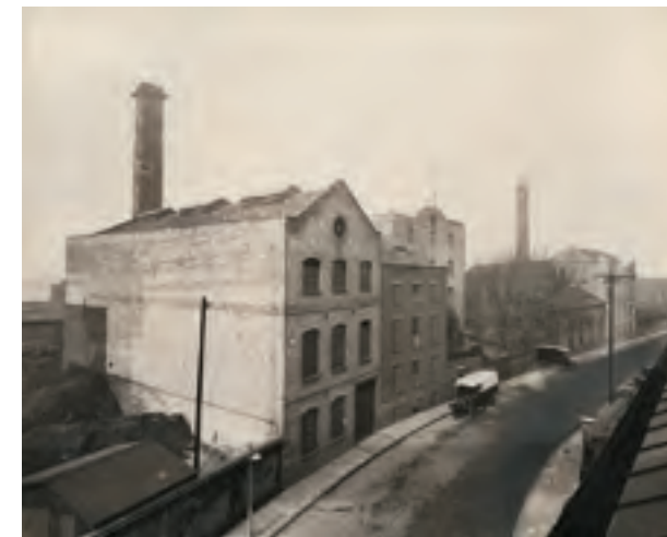
394. Whiffen & Sons' chemical works, Lombard Road, from the south-east, c.1915. Demolished
