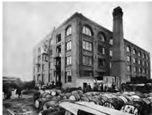
376. T. & W. Farmiloe's warehouse, Nine Elms, in 1885. Demolished
