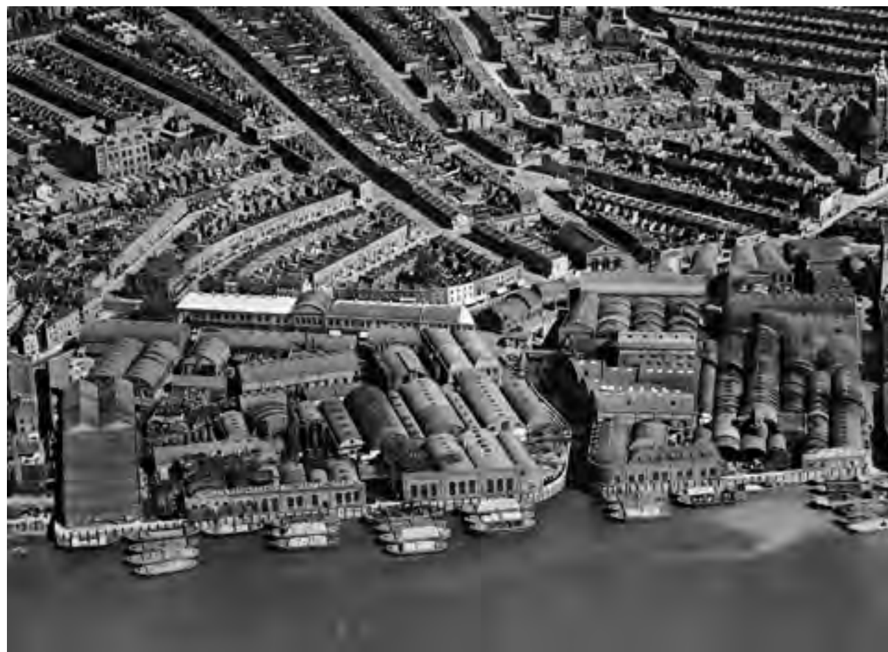
399. Price's factory and York Road area from the air looking south-east, 1928. Mostly demolished
