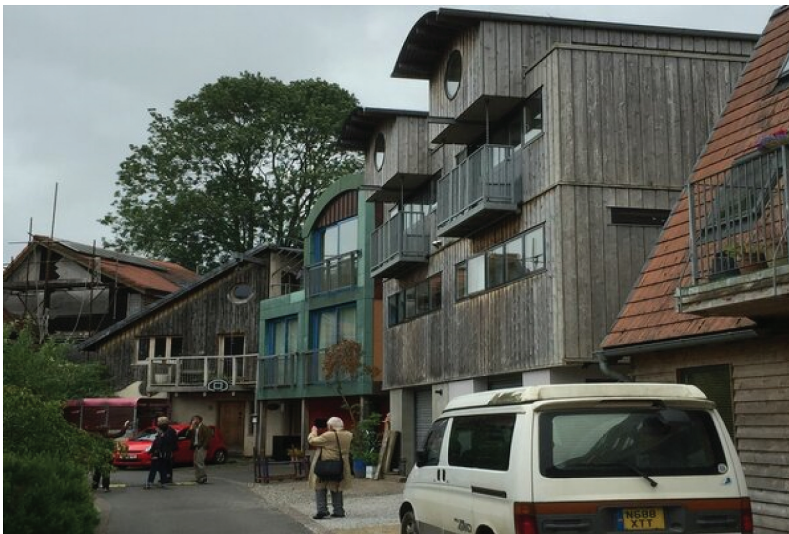
Figure 2. Ashley vale community self-build scheme.
