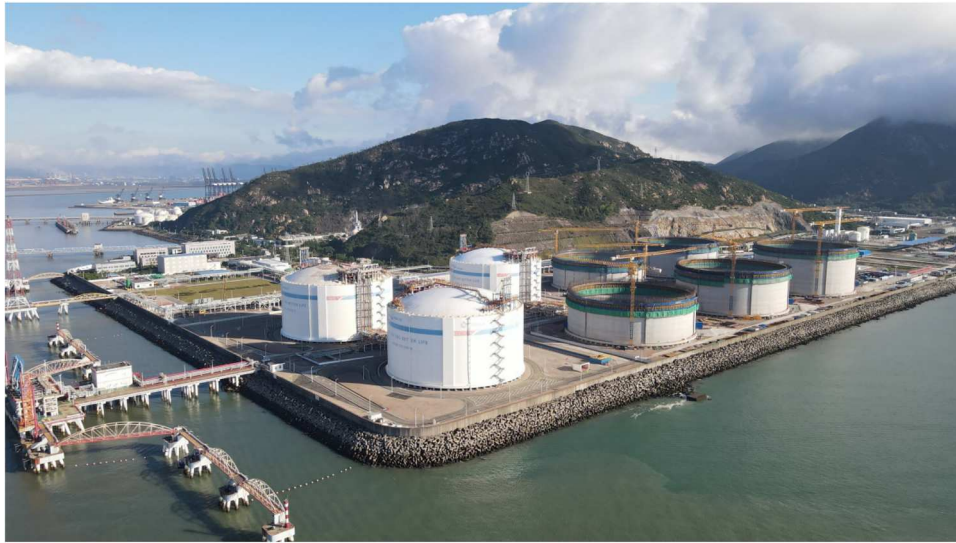
Figure 1. Zhuhai LNG terminal, located in Guangdong Province, China (Zhuhai LNG terminal 2022). (This figure is available in colour online.)
