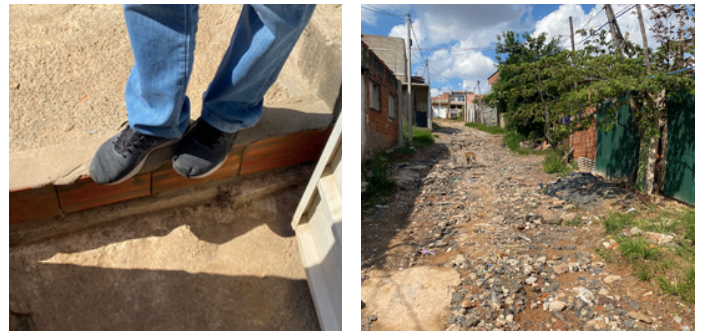
Figure 4: coping strategy to avoid flooding inside the house (left) and street in precarious situation after heavy rain (right).
