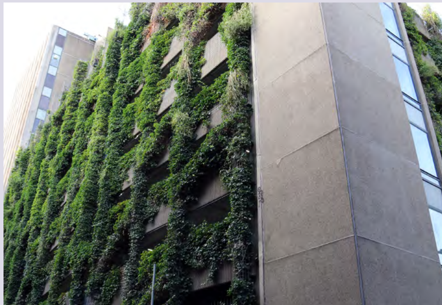
Figure 3. A green wall in Rotterdam, the Netherlands, illustrates DRR in absorbing air pollution. The viewer requires prior knowledge of pollution’s impacts 13 to understand this DRR contribution. The image does not show an unintended consequence: that during droughts the vegetation dries up and can be a major fire hazard for the building.
