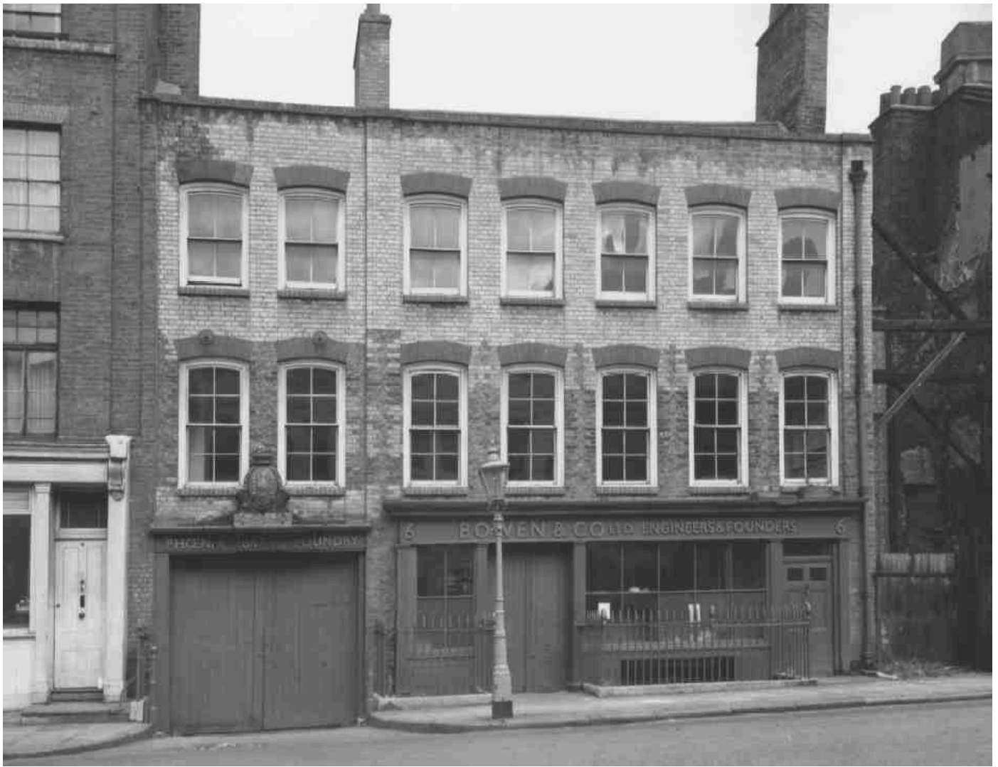
27. No. 6 Mount Pleasant, part of Bowen & Co.'s Phoenix Brass Foundry, in 1965. Demolished
