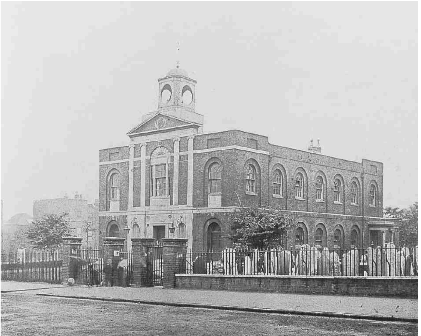
455. St James's Church, Pentonville. View from south-east, c.1900
