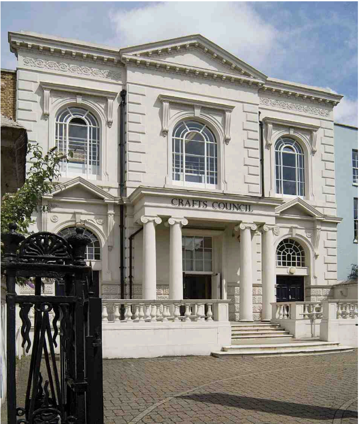
444. Former Claremont Chapel, No. 44a Pentonville Road, in 2007
