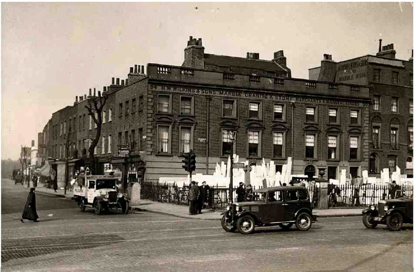
446. Nos 90–94 Pentonville Road, Wilkins' marble works, at the corner with Penton Street, c. 1930. Demolished
