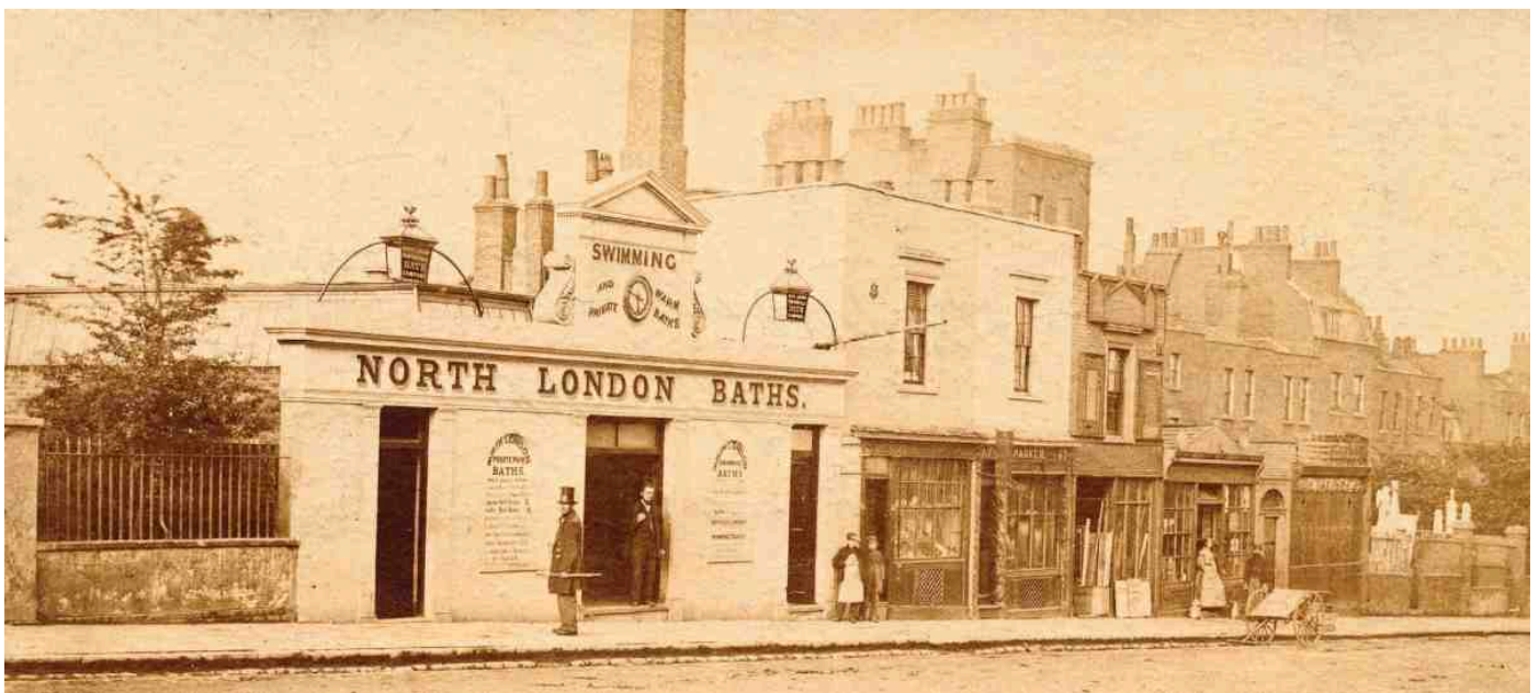
472. Entrance to North London Baths and part of Queen's Row, c. 1863–5. All demolished
