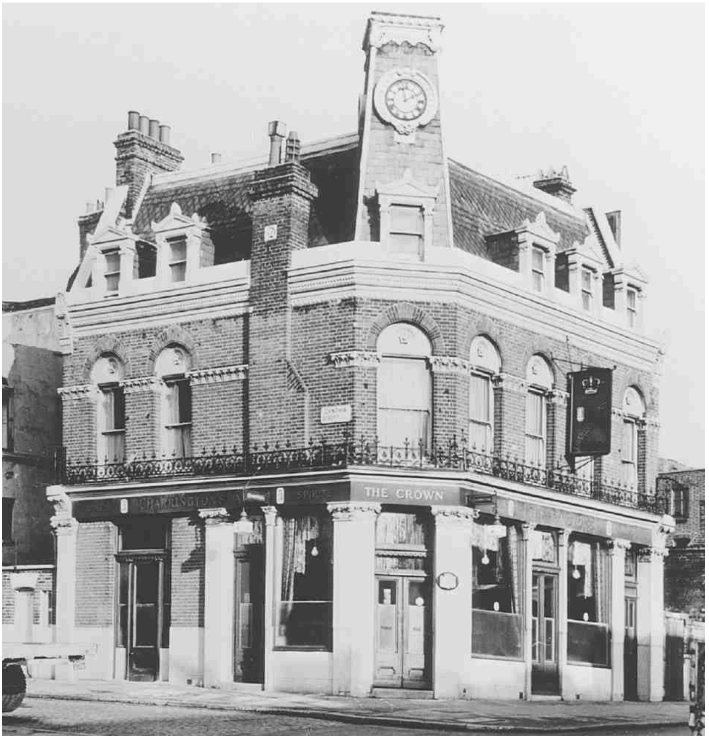
437, 438. Pentonville Road pubs: Lord Vernon Arms, No. 188 (left), rebuilt 1901; Crown, No. 128a, rebuilt 1873–4. Both demolished
