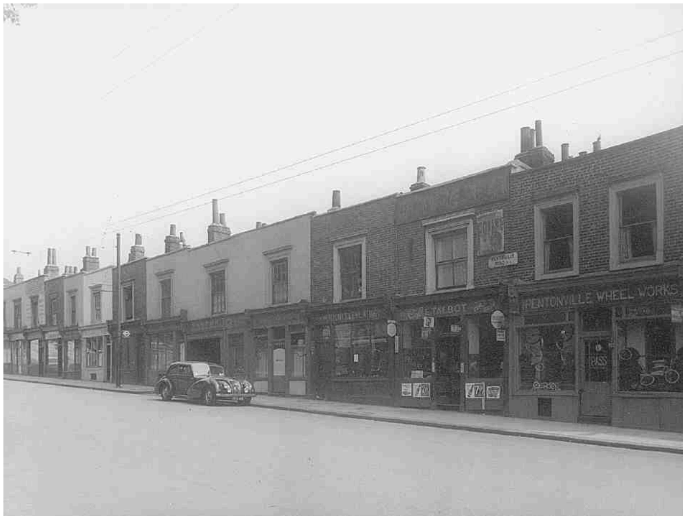
474. Part of former Lower Queen's Row, Nos 151–175A Pentonville Road (left to right), in 1959. Demolished
