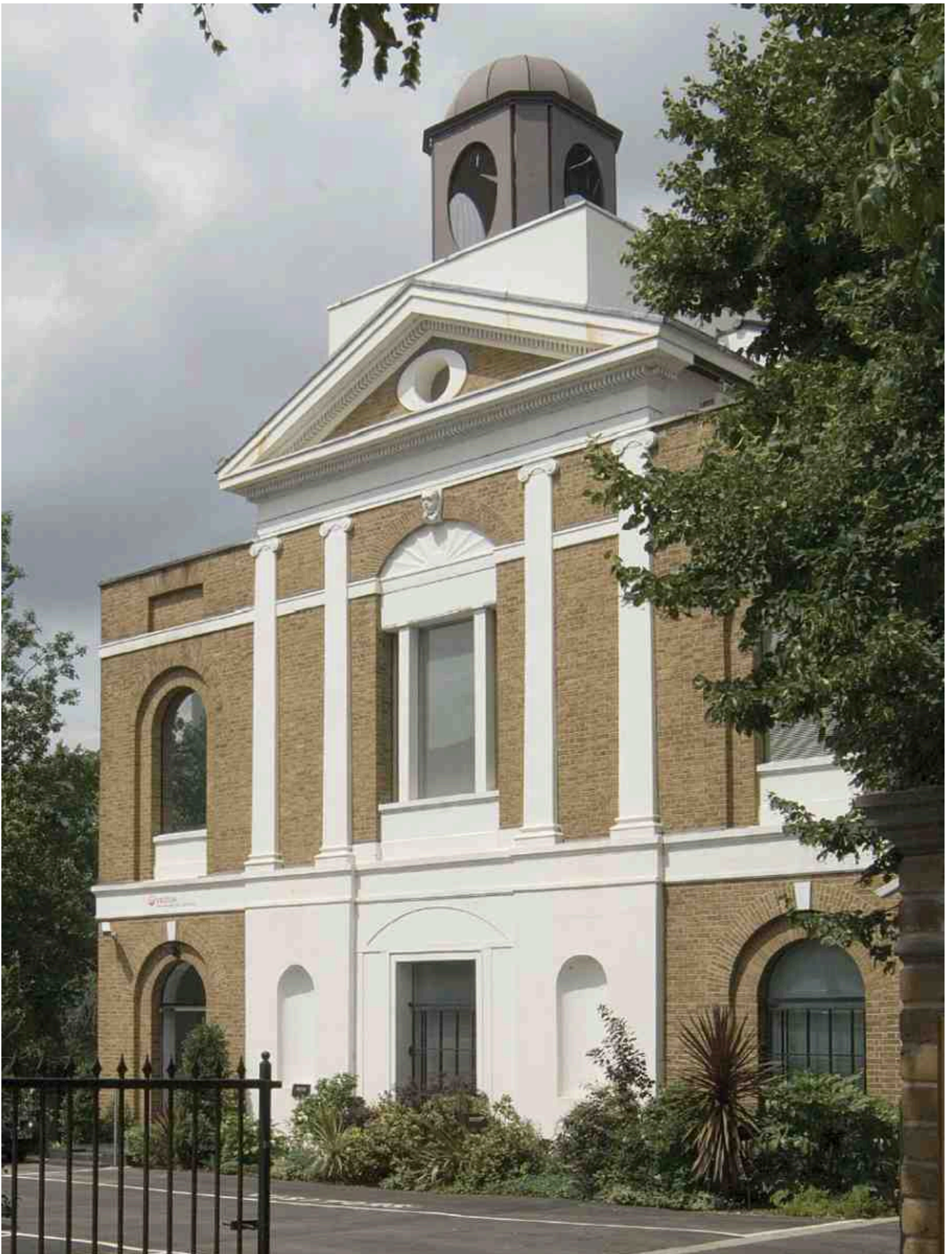
459. Grimaldi Park House, Pentonville Road, in 2007. Allies & Morrison, architects, 1990
