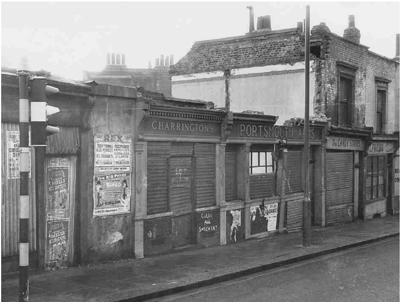
476. Part of former Lower Queen's Row, Nos 139–149 Pentonville Road, in 1963. Demolished
