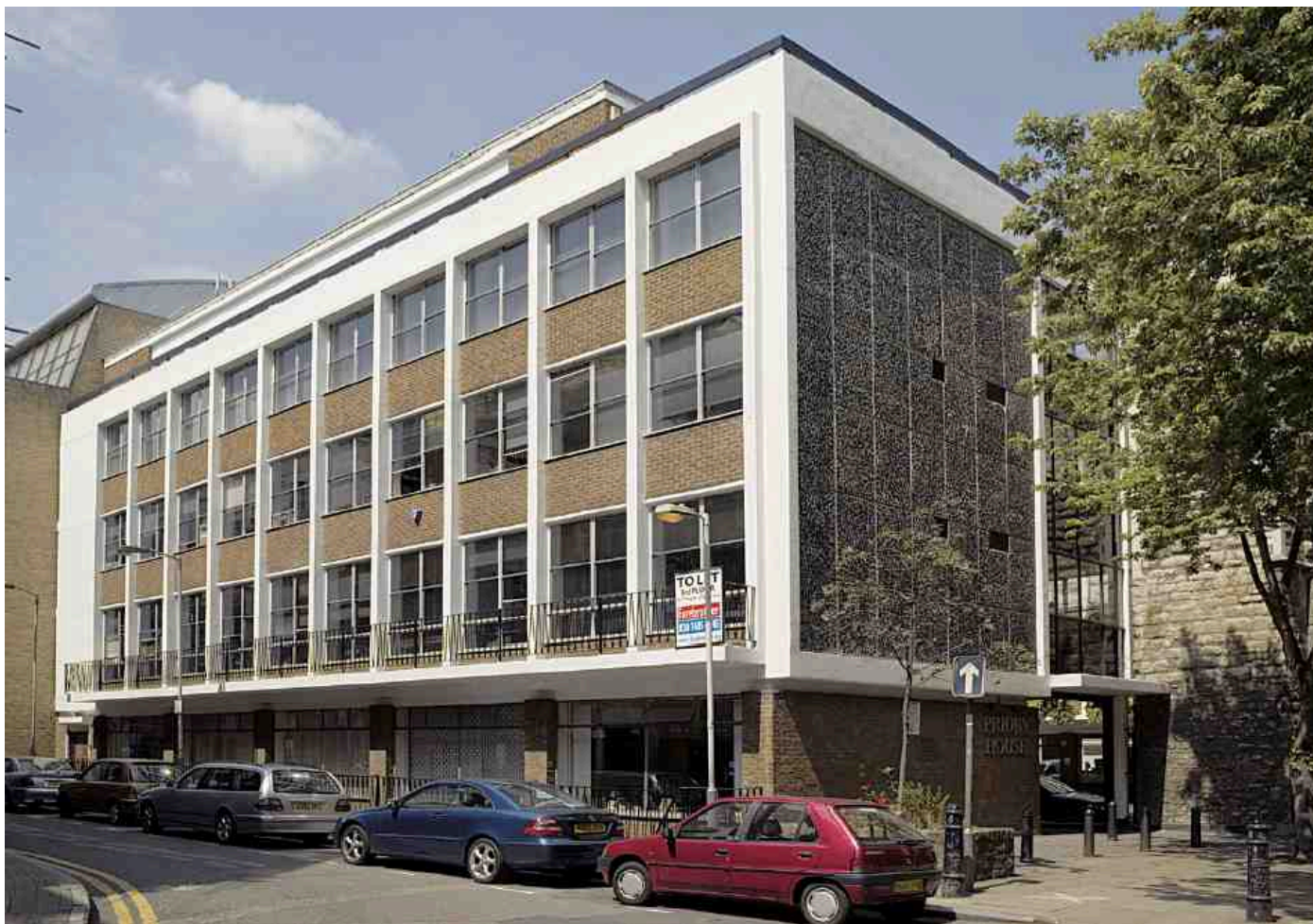
202. Priory House, St John's Lane frontage, 2006. Alec Shickle, architect, 1960–2
