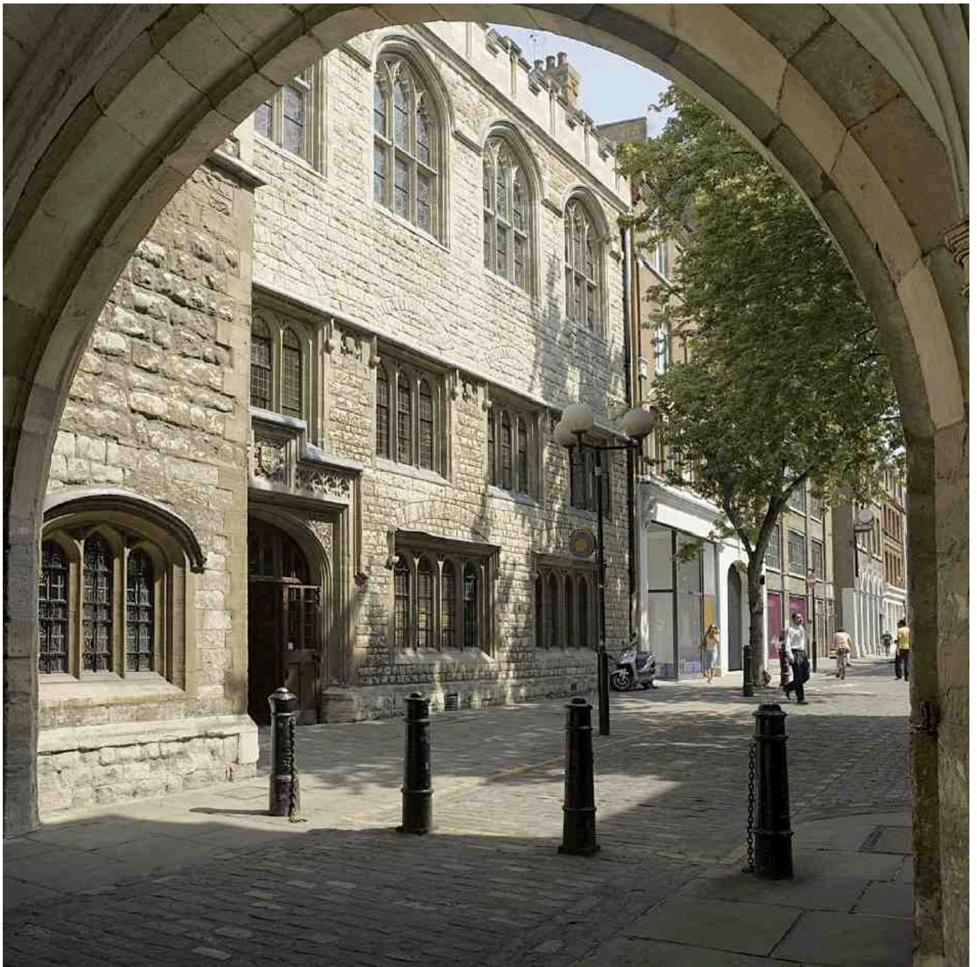
192. St John's Gate. Chapter Hall extension in 2006. J. Oldrid Scott, architect, 1899–1903
