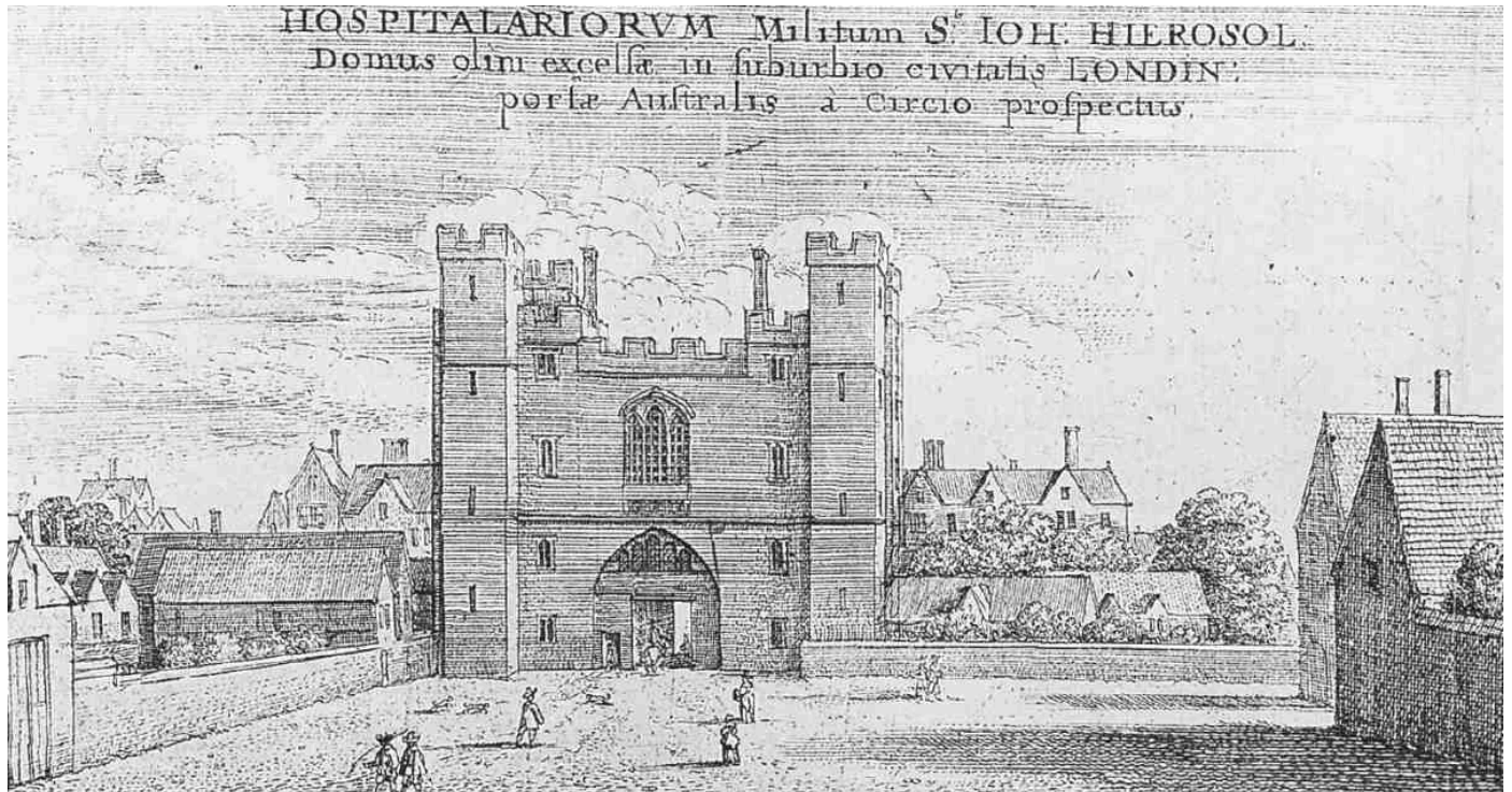
178. St John's Gate, north front, c. 1661. Behind the gate to the right is Berkeley House
