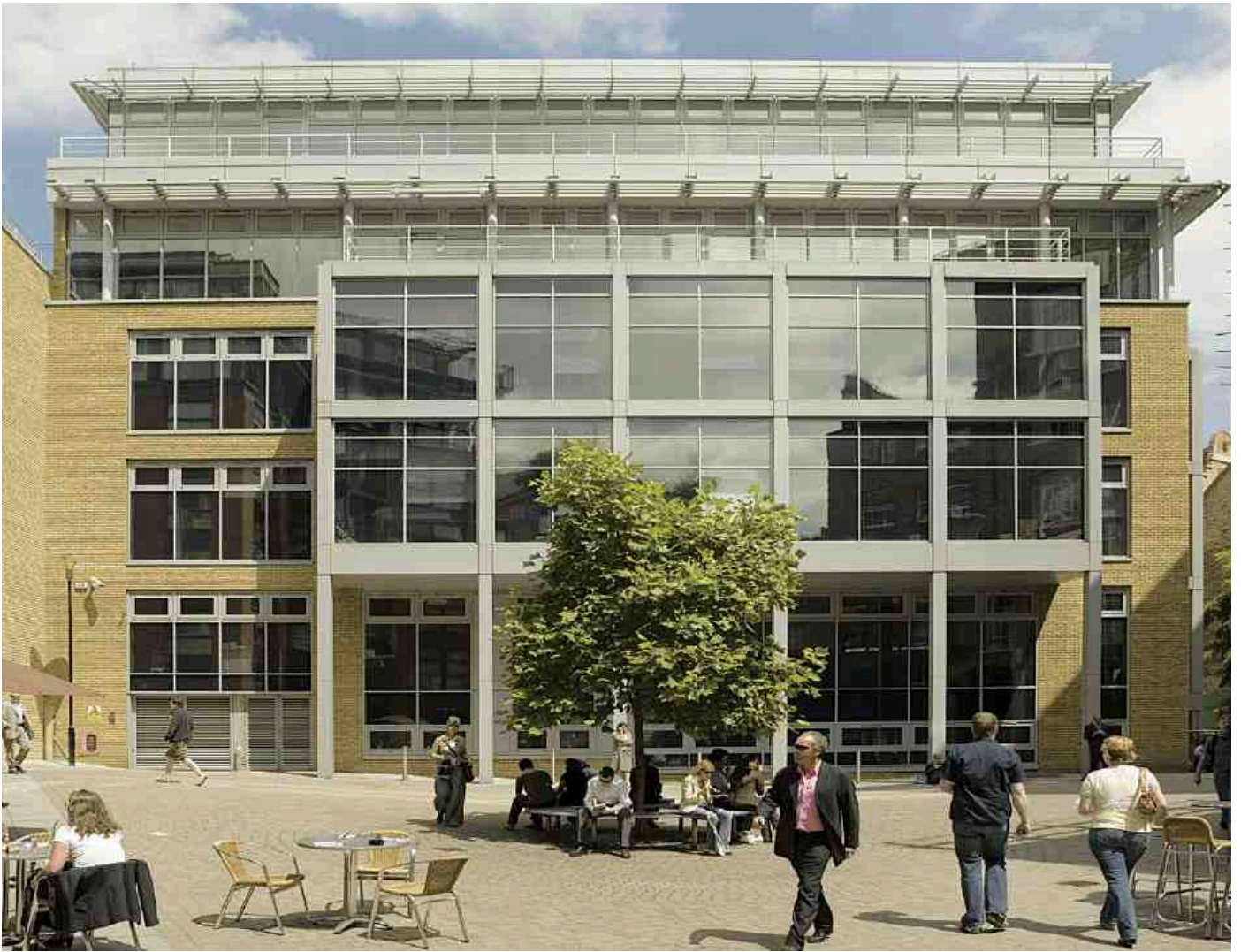
200. Exchange Place, No. 1 St John's Lane, in 2006. The Thomas Saunders Partnership, architects, 2001
