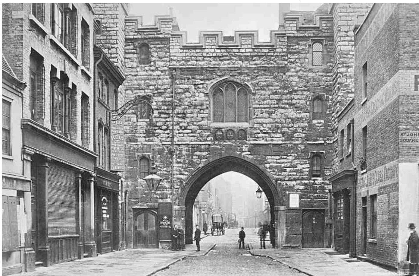
186. St John's Gate, north front, late 1880s; after J. Oldrid Scott's restoration of the Council Chamber over the arch, but before the replacement of W. P. Griffith's battlements
