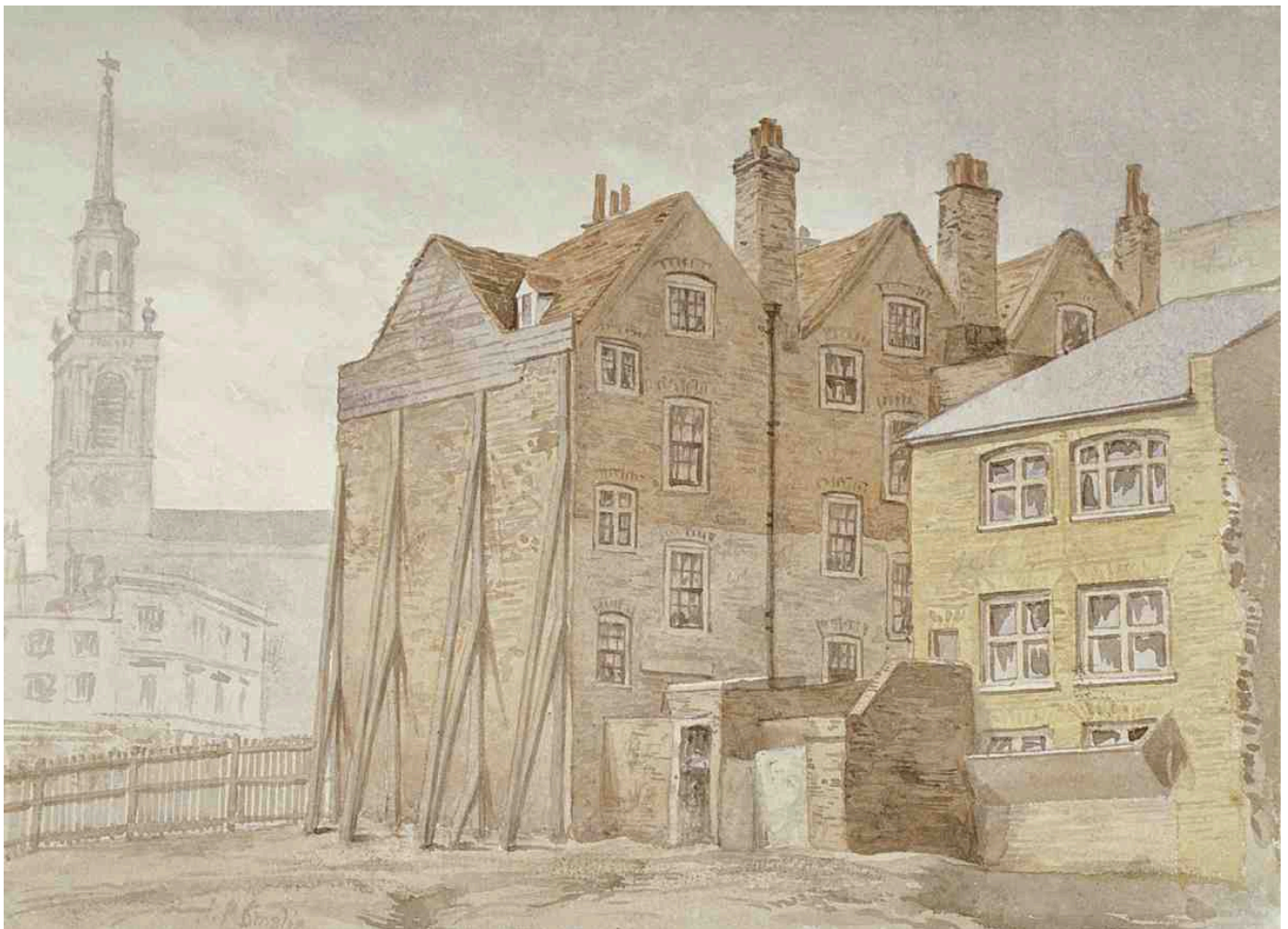
118. Nos 15–17 Clerkenwell Green. Rear view in 1880, following clearance for Clerkenwell Road.
