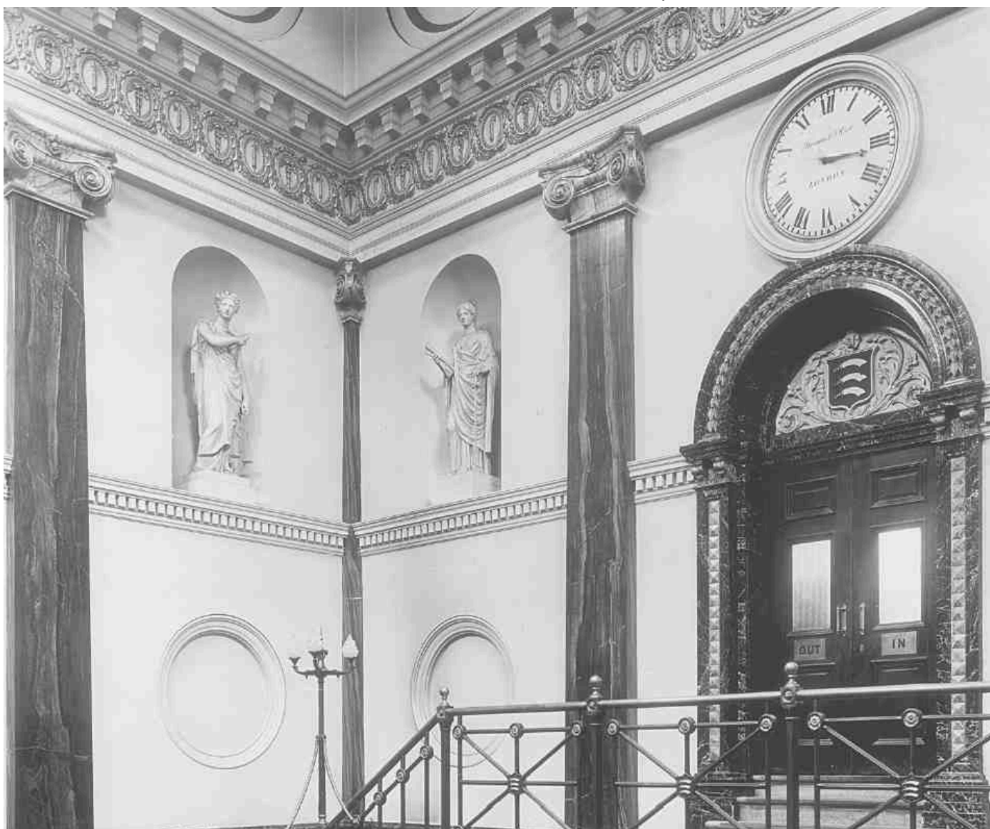
112. Middlesex Sessions House, entrance hall, 1914. East end, showing door to second court-room, and statues by Domenico Brucciani, both of 1859–60
