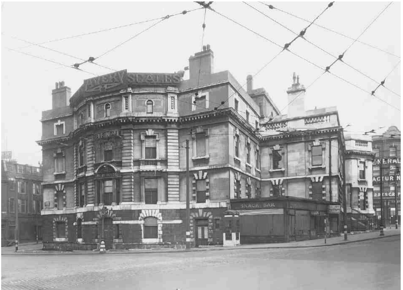
114. West front in 1945, showing additions of 1859–60 and single-storey shops on the site of prisoners' entrance
