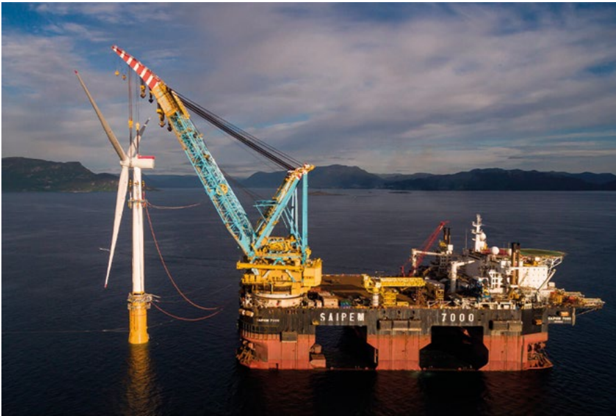
Picture 3. Off-shore wind farm installed by Saipem in Scotland.
