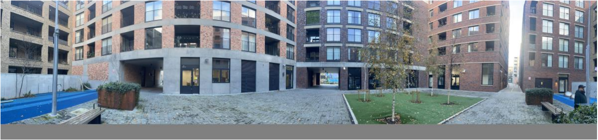
Figure 3. Panoramic Photo of Sensor at Courtyard.
