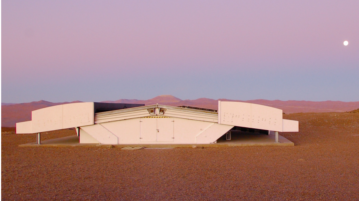
Figure 1. The NGTS enclosure during dusk moon-rise at ESO's Paranal Observatory in Chile. The roll-off roof is open, allowing each of the 12 telescopes an unobstructed view of the night sky to an airmass of 2.0 ( 60^\circ from zenith). Image credit: D. Bayliss
