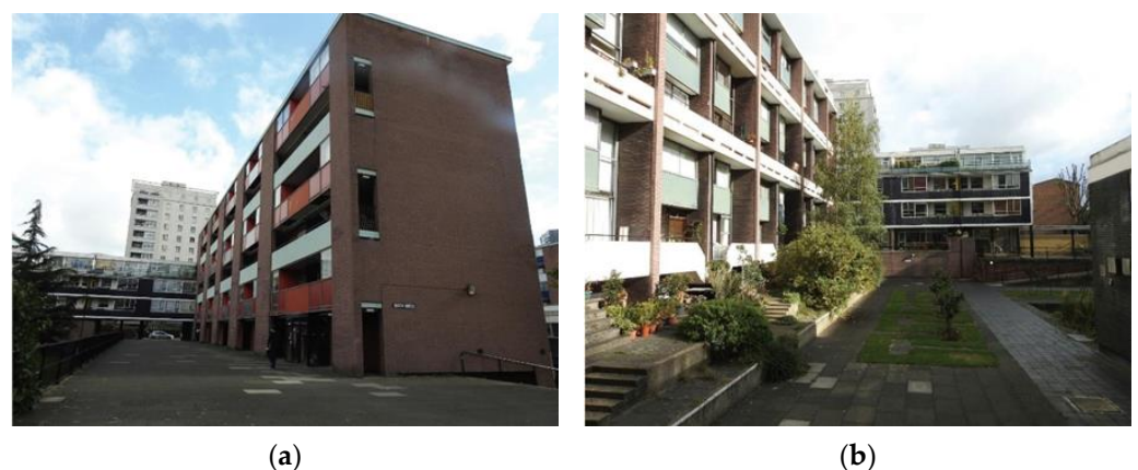
Figure 2. Golden Lane Estate: (a) the Bayer House front façade; (b) the Bayer House south façade and back courtyard (source: Sharmeen Khan, student 2014–15).
