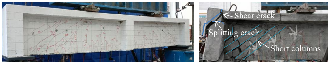
(b-1) Front view of failed beam (b-2) Side view of the failed details
