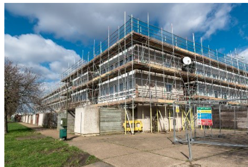
Figure 4. A housing block undergoing refurbishment, mid 2017 (Credit: Richard Timmerman).
