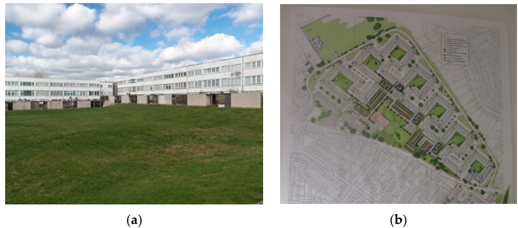
Figure 3. (a) General view of a courtyard, Pollards Hill. (b) Public display poster of Pollards Hill master plan, showing the seven courtyards featured in the project (Credits: Richard Timmerman; project team).
