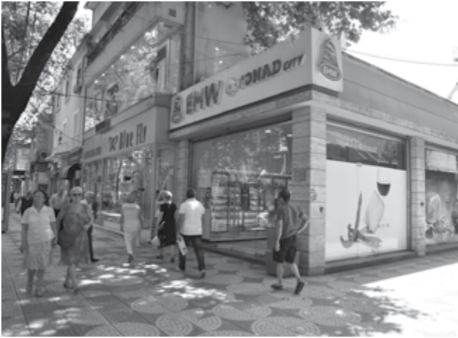
CONVERSION OF LAND USE ON THE GROUND-FLOOR LEVEL, FROM DOMESTIC TO NON-DOMESTIC, ALSO EXTENSION OF NON-DOMESTIC USE ON THE SIDE OF THE BUILDING (ALTERING ITS ORIGINAL FOOTPRINT)
