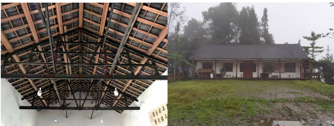
Figure 7. The Internal and External Pictures of the Reconstructed Community Hall.
