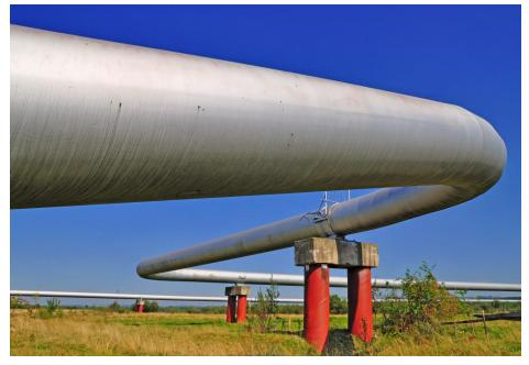
**Gas-phase:** up to 35 bar, 5 to 40 °C **Dense-phase:** 85 to 150 bar, 12 to 44 °C
