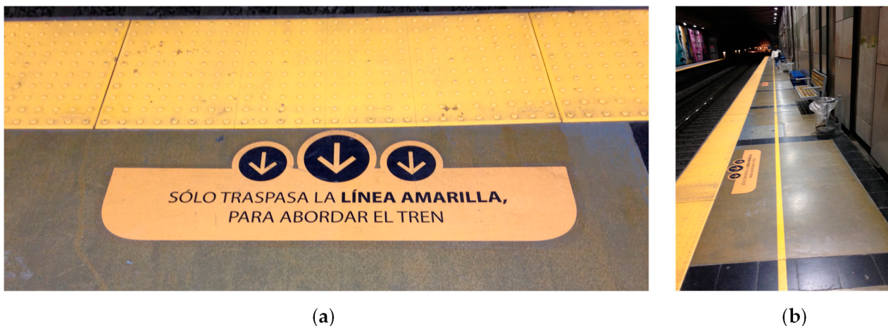
Figure 3. Yellow safety line observed in metro stations in the Valparaiso Metro, Chile: (a) 60 cm width (carbon and fiberglass reinforced with yellow pods) used with the marking “only cross the yellow safety line when boarding the train” and (b) the yellow safety line is used with another yellow line in the middle of the platform to encourage movement on the right-hand side and prevent passengers walking next to the platform edge.
