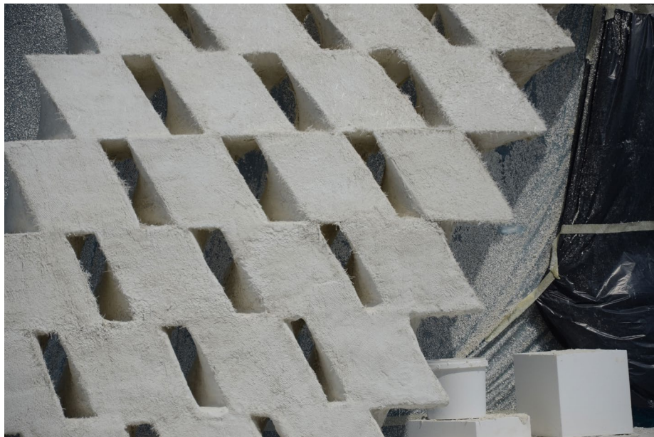
Fig. 12. The application of GRC on the final prototype.
