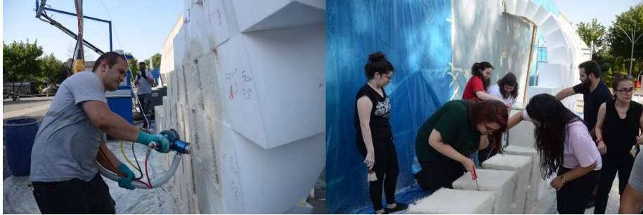
Fig. 16. Application of GRC on stay-in-place form-work.
