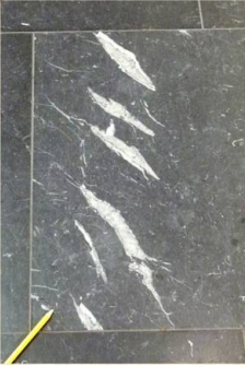
Tension cracks
