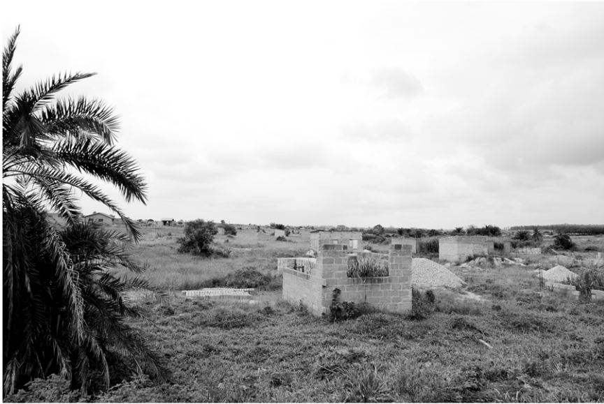
Figure 1. Concrete blocks, made up of sand, water and cement, in plots of land, Greater Accra region.
