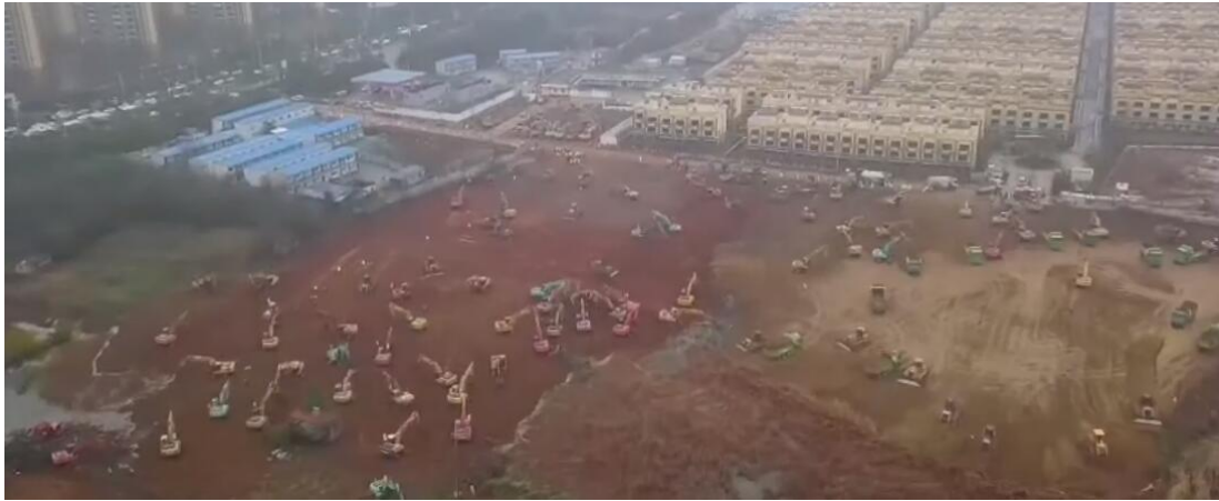
Figure 28 Construction site of Huoshenshan Hospital
