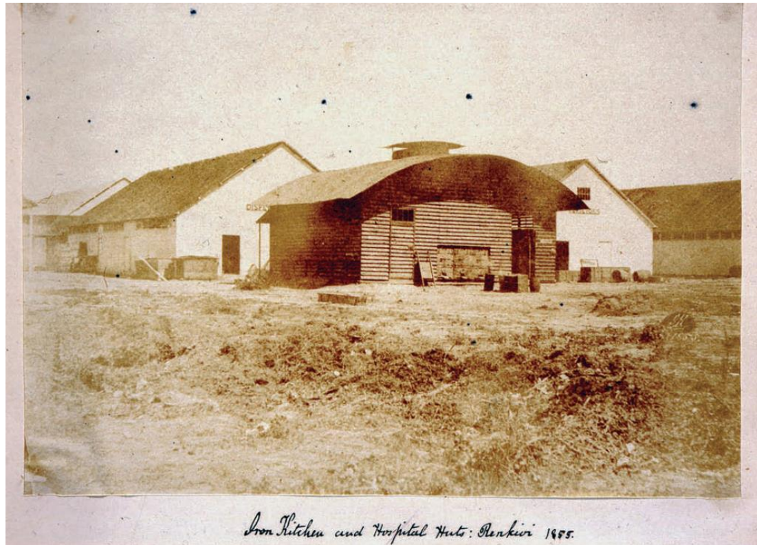
Figure 2 Brunel's revolutionary off-site hospital built in 1855
