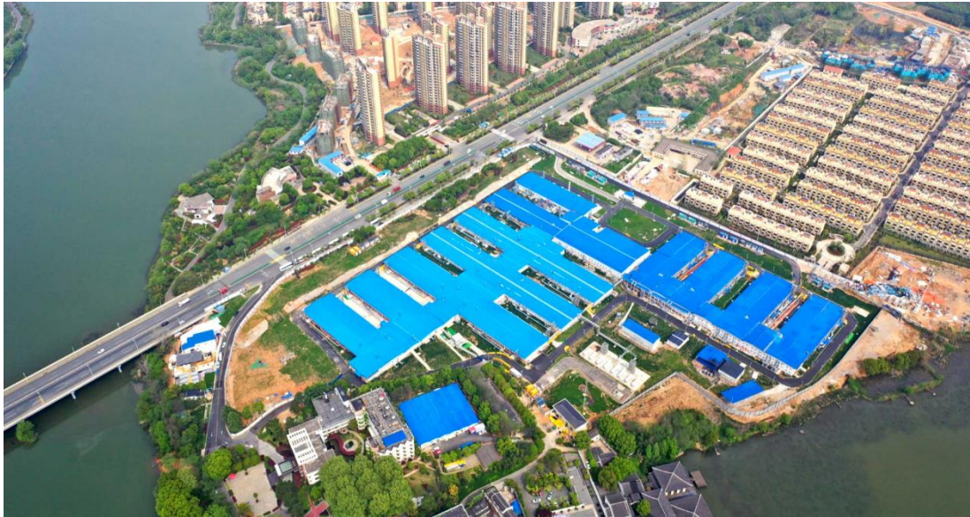
Figure 29 Completion of Huoshenshan Hospital (source: CITIC)
