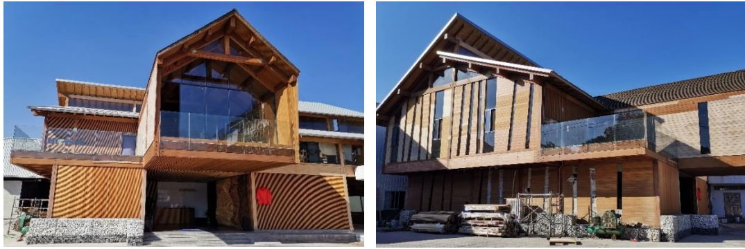
Figure 1 LBL office building (reproduced with permission of Haitao Li)
