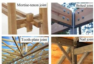
(b) Common wood construction joint types (Source: https://image.baidu.com/)
