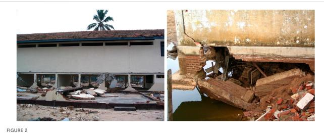
(A) Washed away building in front and washed away infills at the rear. (B) Foundation scouring of a corner.
