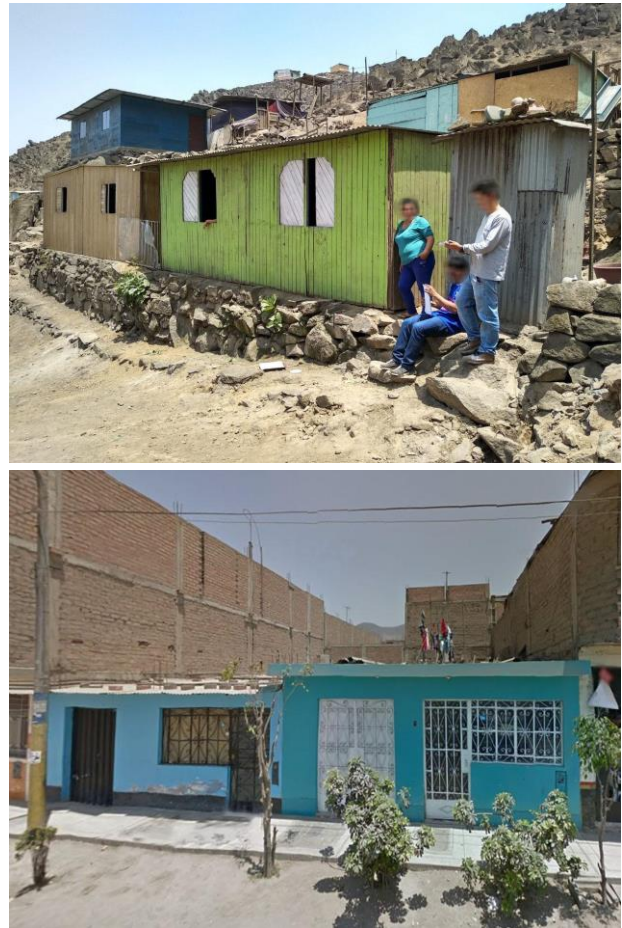
Figure 3. View of housing archetypes: wood (light archetype, upper) and brick (intermediate and substantial archetypes, lower).
