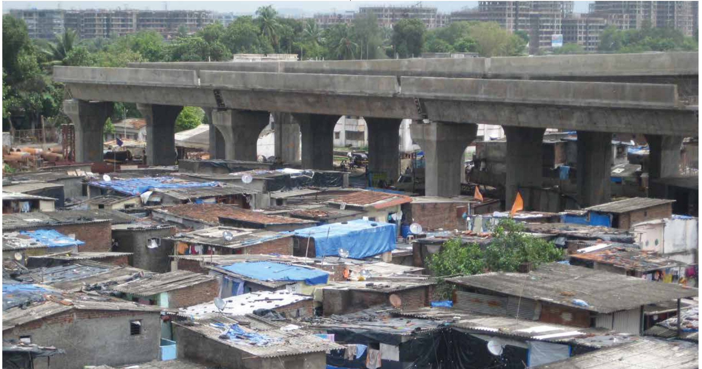
Double-decker flyover at Kurla Terminus.
