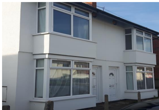
Figure 1. Front elevation (facing S-SE) of the test houses (the left hand house was used in this study).
