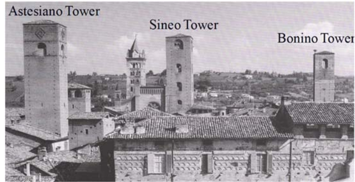
Figure 10: Three medieval towers rising in the center of Alba, that were investigated with AE monitoring. Figure adapted from [16].
