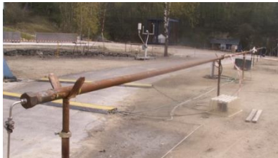
Photograph of the 40 m long, 40mm internal diameter pipeline for conducting the CO 2 blowdown experiments at INERIS
