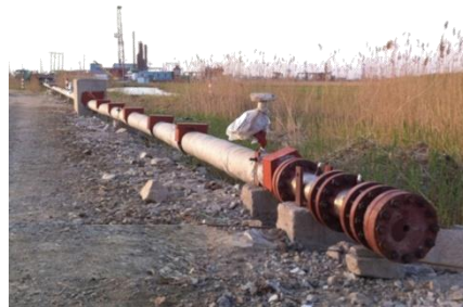
The fully instrumented 256 m long, 0.233 m i.d. pipeline for CO 2 release experiments, constructed by DUT in the Liaohe Oilfield in China
