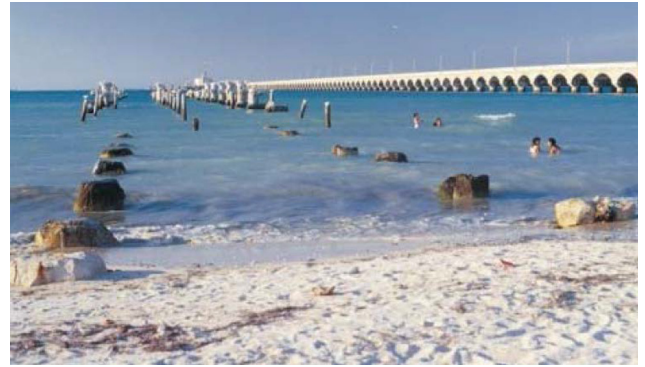
Fig. 1. The Progresso Pier in Mexico [21].
