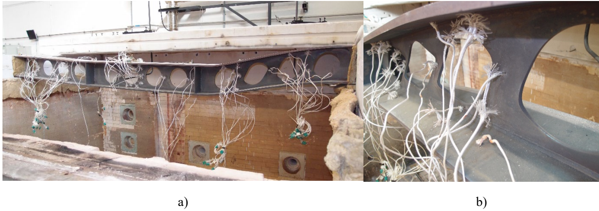
Figure 4: Cellular beam specimen after fire test: a) Steel beam after testing; b) Web post buckling failure mechanism
