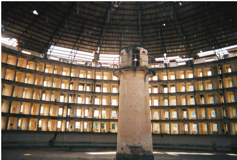
Figure 6.1 Inside one of the prison buildings at Presidio Modelo, Isla de la Juventud, Cuba. The prison consisted of five six-storey structures. The Castro brothers were held here between October 1953 and May 1955. Now a museum and national monument. https://commons.wikimedia.org/wiki/File:Presidio-modelo2.JPG (accessed 31 March 2022). © Friman. CC BY-SA 3.0.
