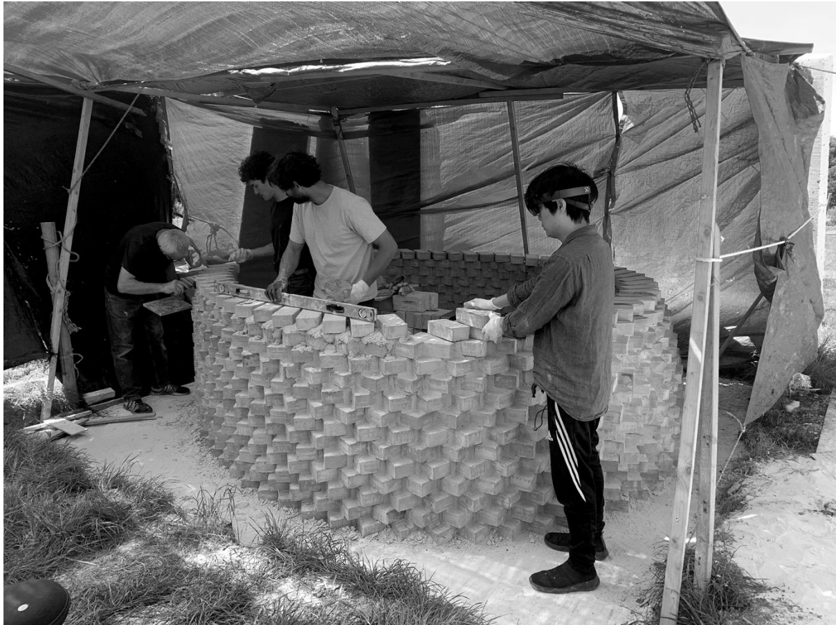
Figure 07: The bricklayer with the HoloLens is in constant dialogue with the team
