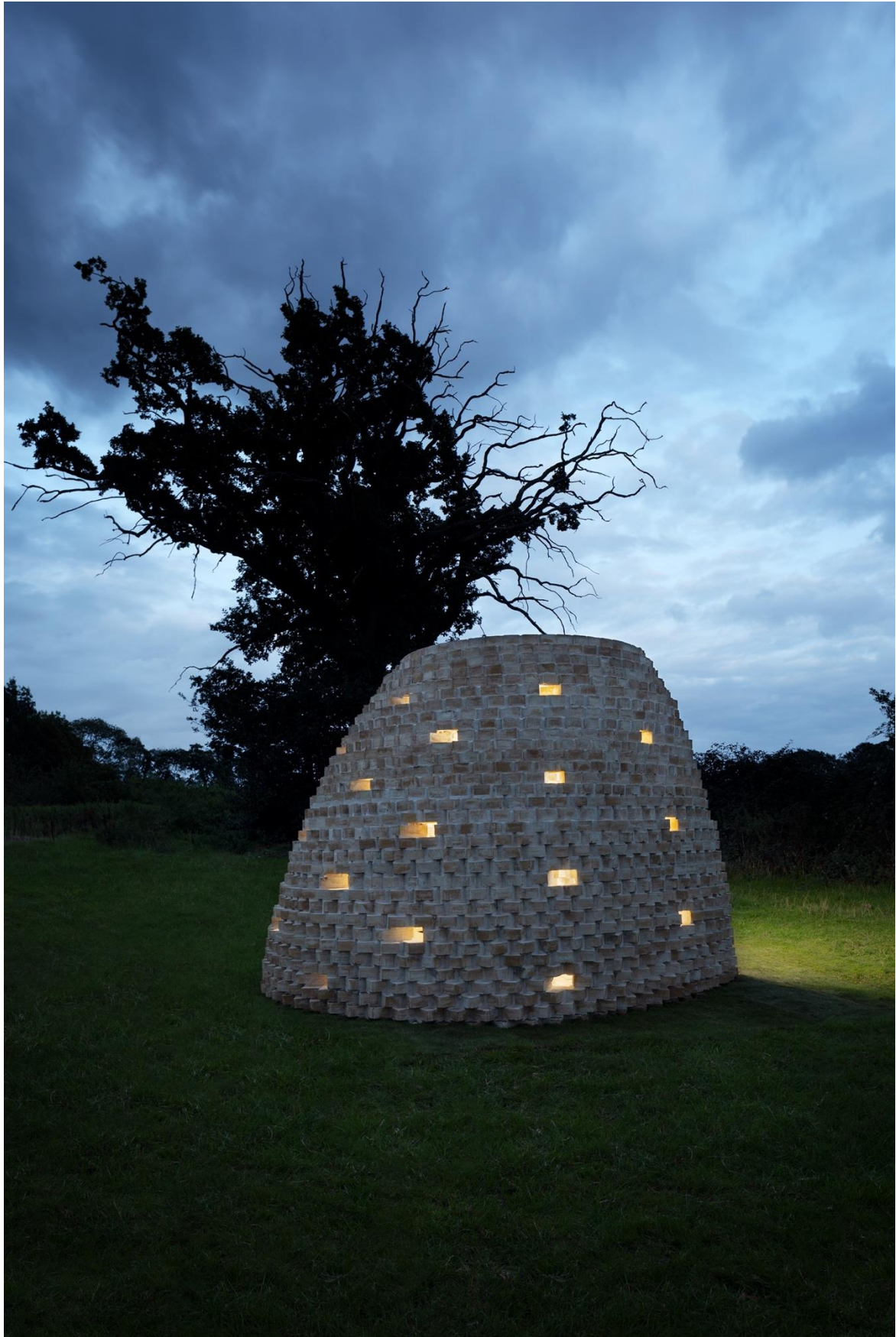
Figure 18: Night view of the Bothy at Grymsdyke Farm
