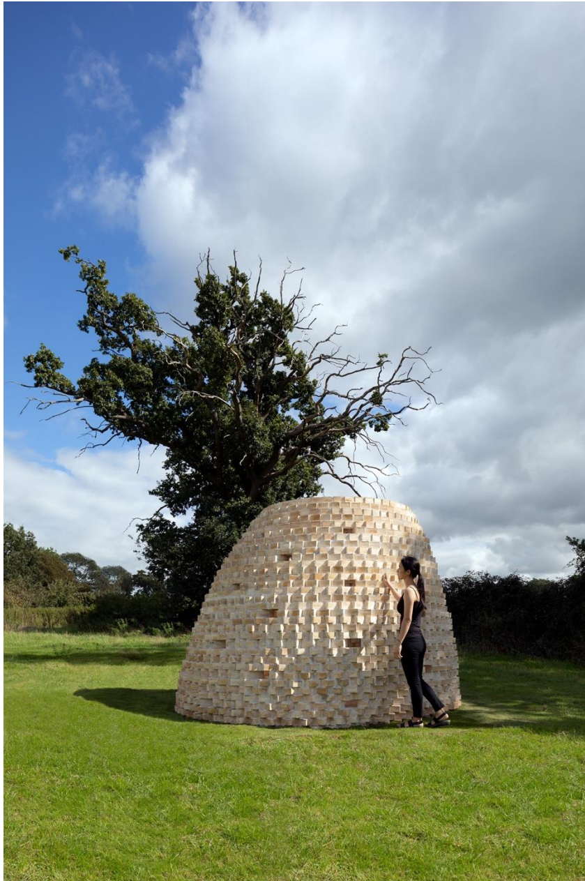
Figure 15: The subtle angle change of the brick arrangement is highlighted with direct sunlight
