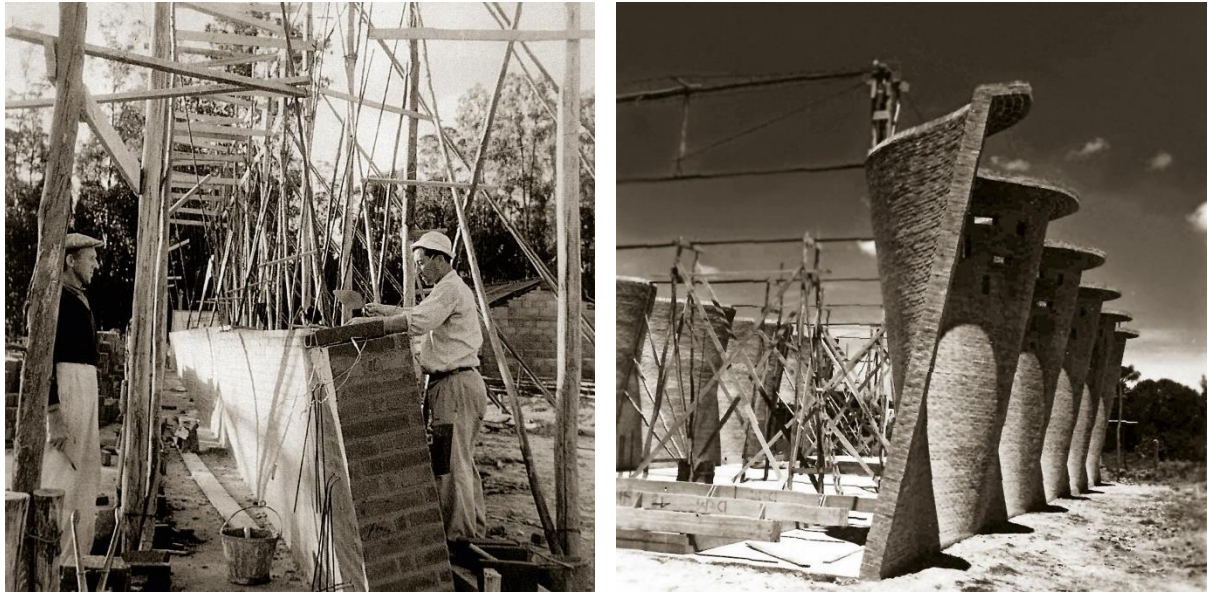
Figure 04: Eladio Dieste's undulating Cristo Obrero Church under construction, © Universo C eramico ( https://arquitecturaviva.com/articles/eladio-dieste-100-years )
