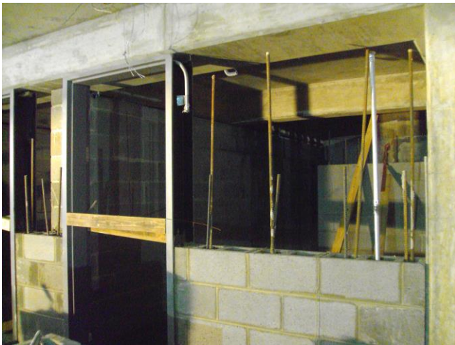
FIGURE 3 Difficult Wall (Wall Difficulty=3). Picture by L. Florez-Perez.
