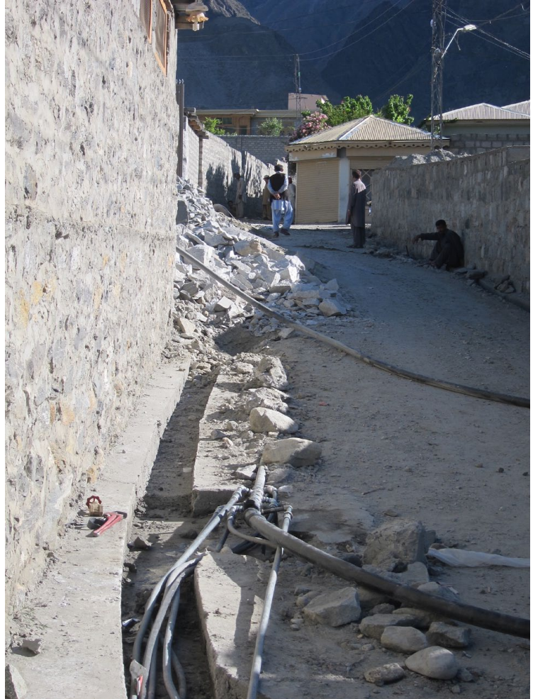
PHOTO 2 Laying of WASEP pipes in Ameenabad, Gilgit
