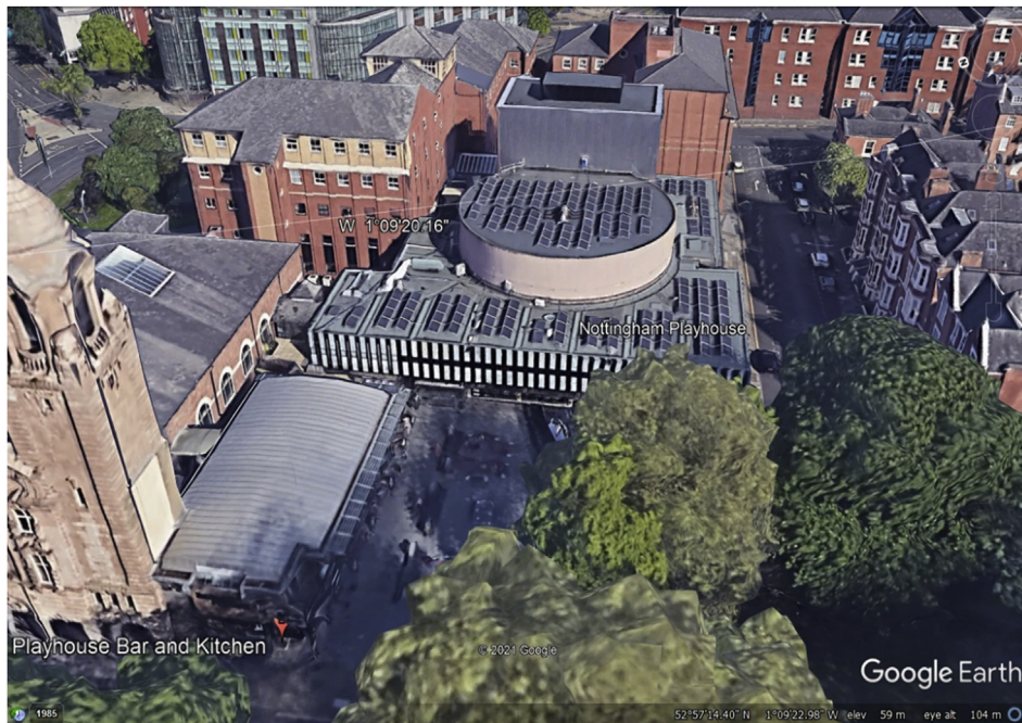
Fig. 25 Post-retrofit Nottingham Playhouse with the photovoltaic solar panels on the roof (Credit: Google Earth, under Geo Guidelines).
