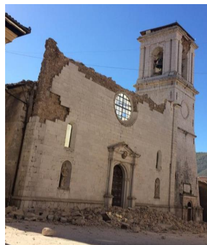
Fig. 1 Out-of-plane damages caused by earthquakes to monumental buildings: a) Christchurch (NZ) 2011, b) Norcia (IT) 2016.
