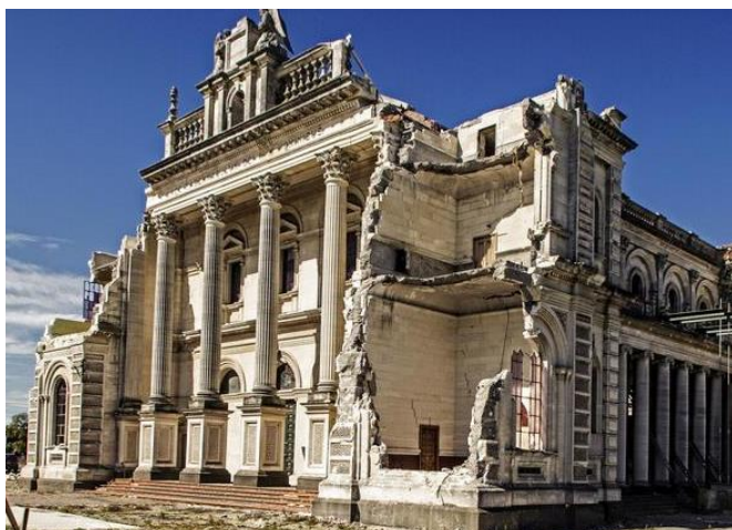
Fig. 1 Out-of-plane damages caused by earthquakes to monumental buildings: a) Christchurch (NZ) 2011, b) Norcia (IT) 2016.
