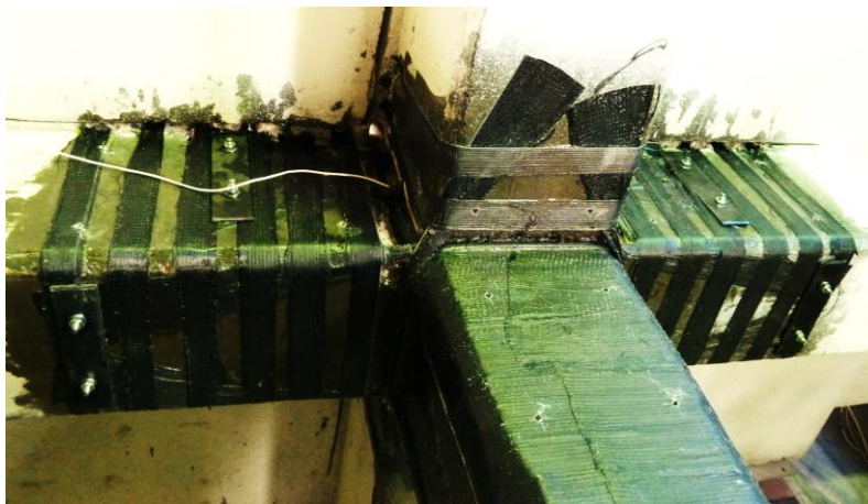
208 209 Fig. 2. Retrofit applied to a specimen with slab and transverse beams. 210
