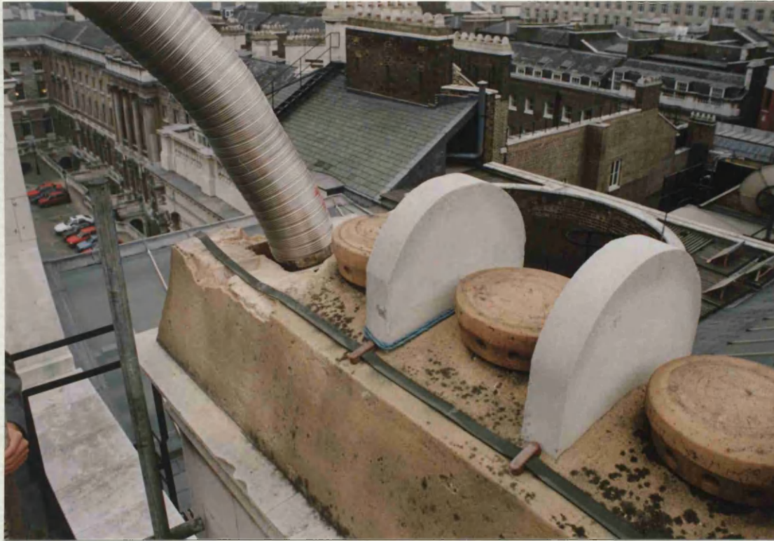
Plate 9: Ductwork being used to line the chimney flues at Somerset House.
