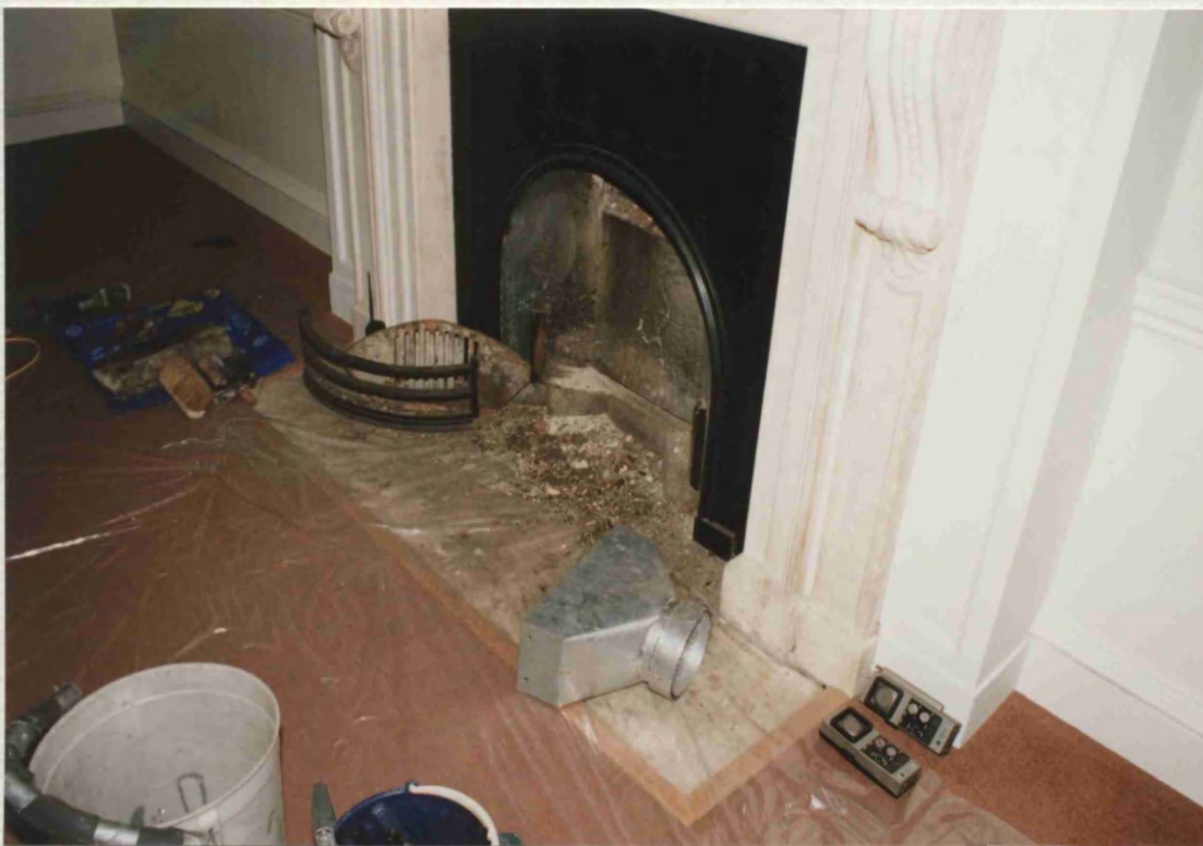
Plate 8: Cleaning the fireplaces at Somerset House in preparation for ductwork.
