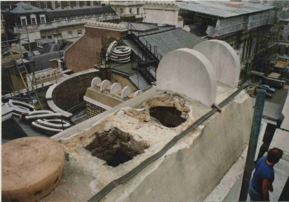
Plate 7: Uncapping and clearing of chimney flues at Somerset House.
