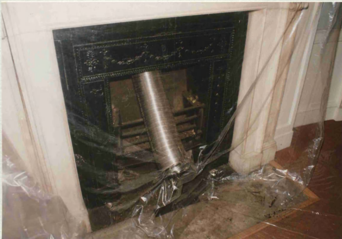
Plate 10: Ductwork emerging into the Galleries via the fireplace.
