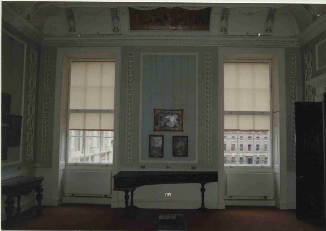
Plate 6: Sealed secondary glazing with integral blind system in windows of Courtauld Institute Galleries.
