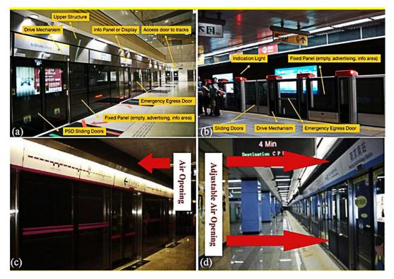
Figure 6: Platform doors in UMSs (a: PSDs; b: APGs; c: PBDs and d: AVPDs).
