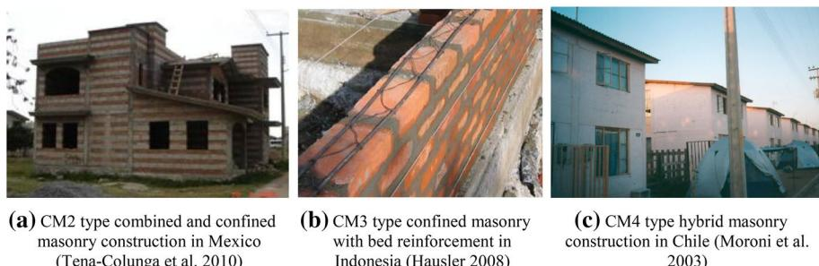
**Fig. 4** CM2, CM3 and CM4 type confined masonry construction
