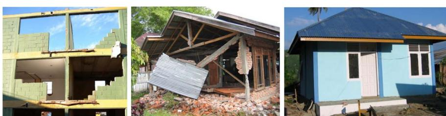
**(a)** Failure of CM walls with no confinement around large openings- 2010 Chile earthquake (Brzev et al. 2010)
