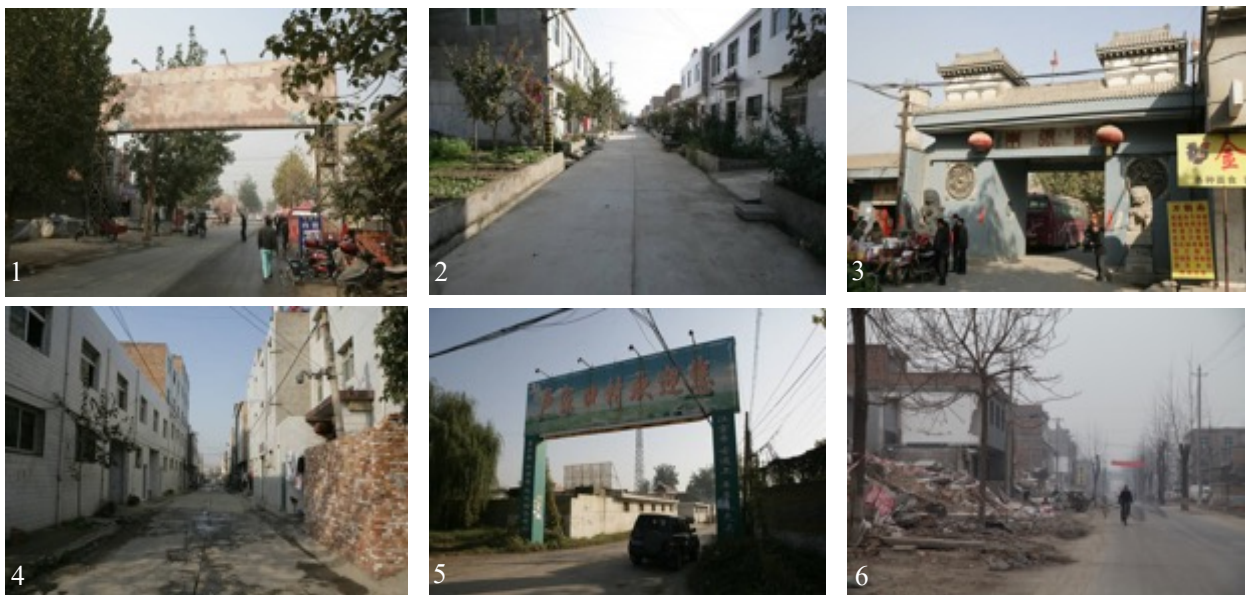
Figure 3. Five of the villages in the site area and the appearance of the street while the removal.
