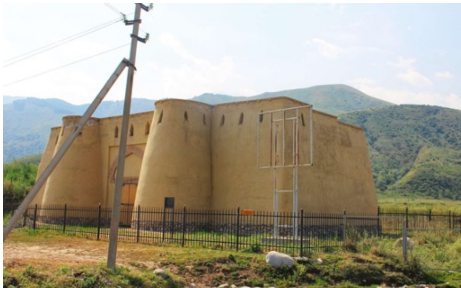
Figure 44 The reconstructed front gate
