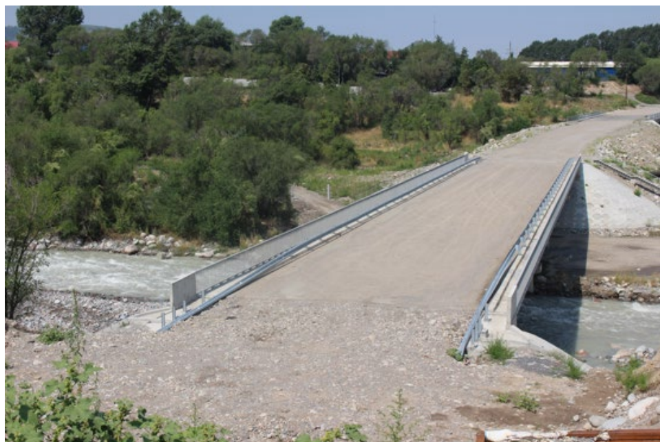
Figure 46 The modern bridge over the Talgar River
