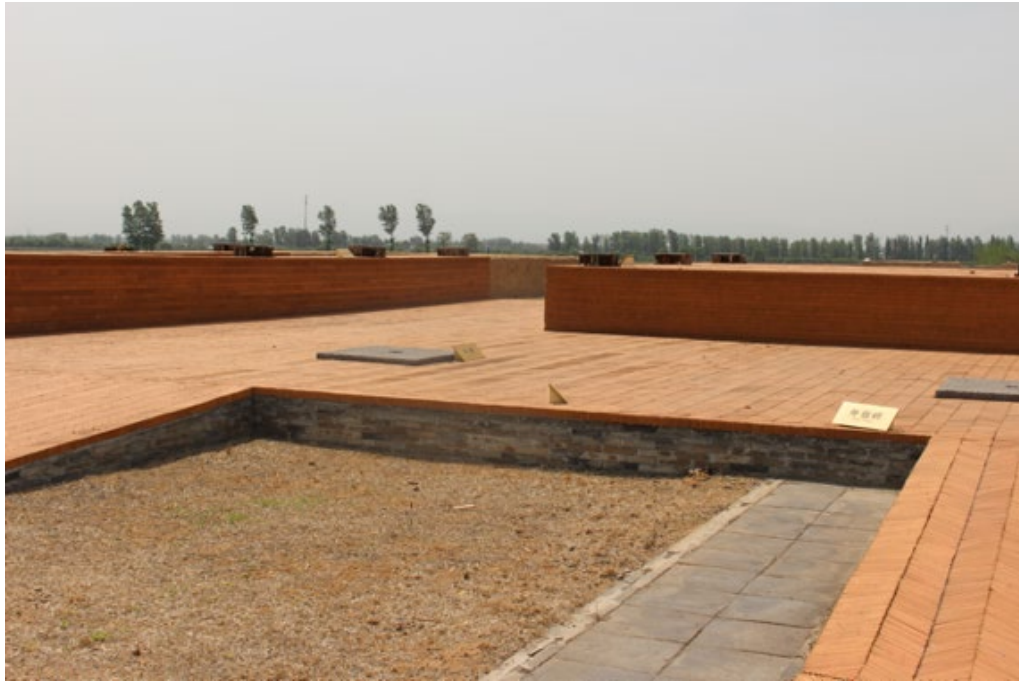
Figure 26 The reconstruction work over the ruins of the side hall
