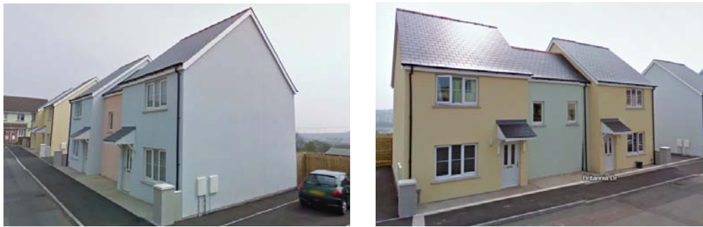
Figure 3: Britannia Drive - south elevation before installation of Photovoltaic panels: south east view (right) south west view (left).
