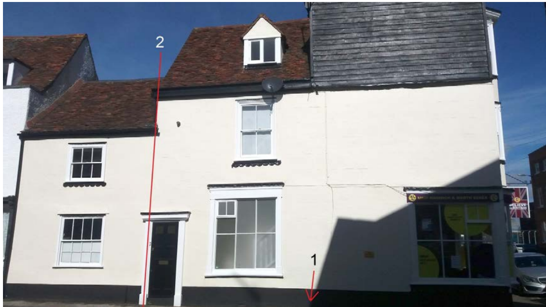
Figure 3: View of the south-east side of the property (site south) showing the approximate position of the north-south partition in the cellar shown in Figure 5 (1) and the line of the east-end gable wall shown in Figure 6 (2) (photograph: Martin Bridge)
