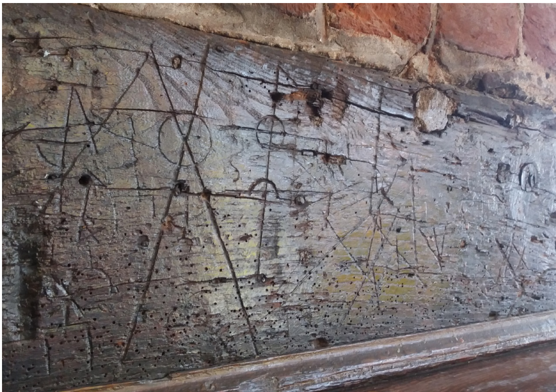
Figure 4: Mantel beam in ground-floor north room (fronting onto King's Quay Street) with an abundance of apotropaic marks, the exposed end of this beam was photographed to derive sequence hsta01 (photograph: Martin Bridge)
