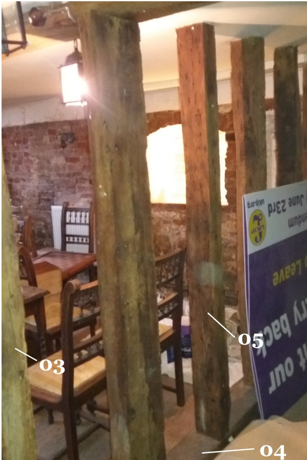
Figure 5: Part of the basement stud wall showing some of the timbers sampled (photograph Martin Bridge)
