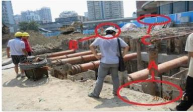
Edges of excavations (over 2m deep) should be protected with a guardrail
