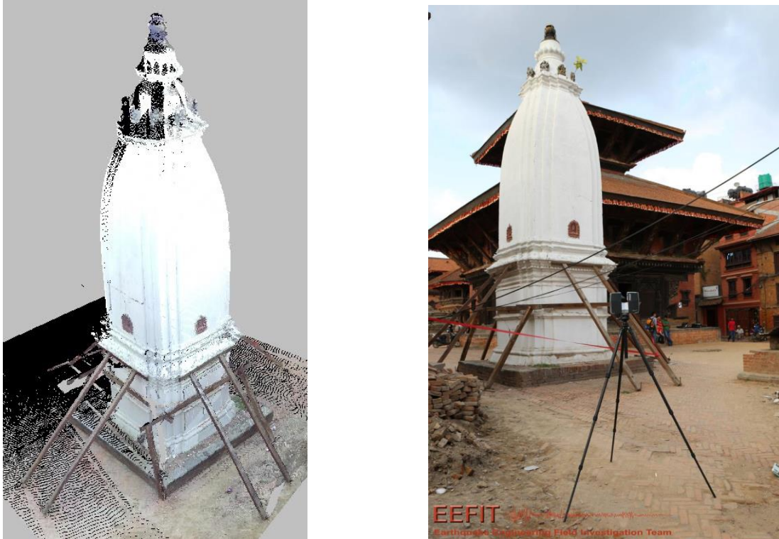
Figure 1. A point cloud of Nepalese temples after the Gorkha earthquake captured using a terrestrial laser scanner and a photographic image of the same
