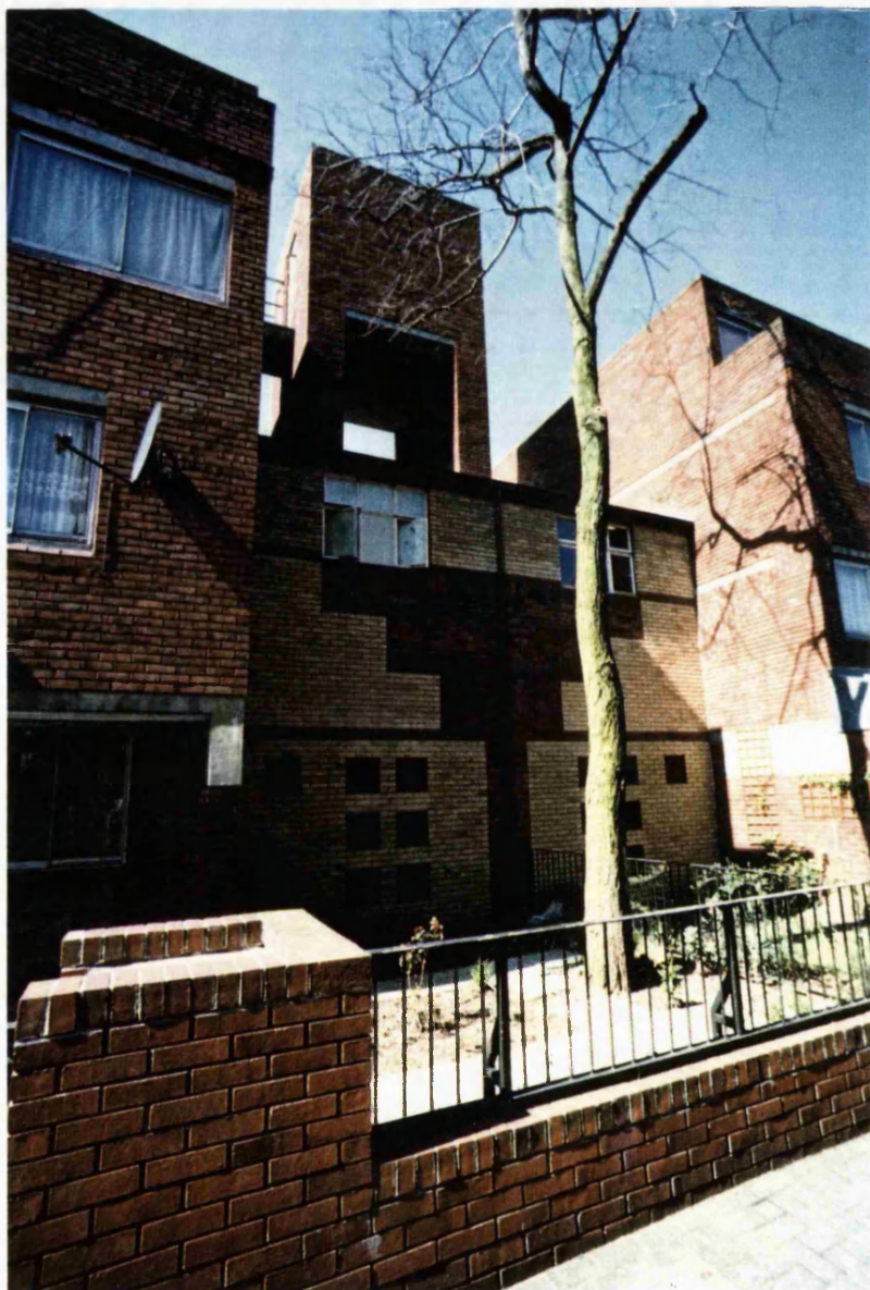
Plate 35: The back of the stairwell as viewed from Parry Road.
