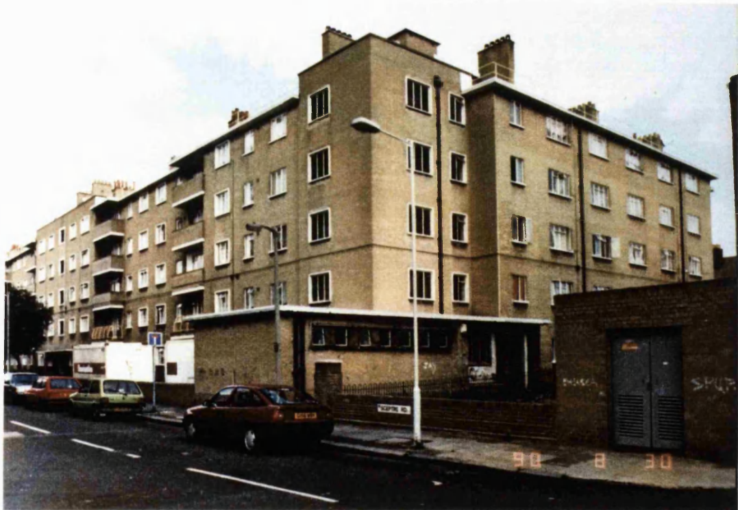
Plate 52: A view of the block prior to refurbishment from Sceptre Road.
