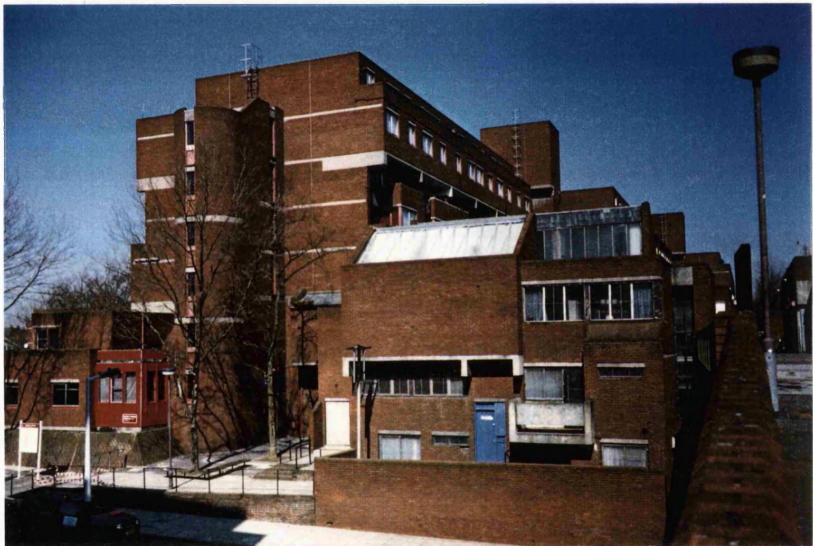
Plate 1: Onslow House as seen from the central walkway, it is a large block and is attached to the walkway and to Severn House.
