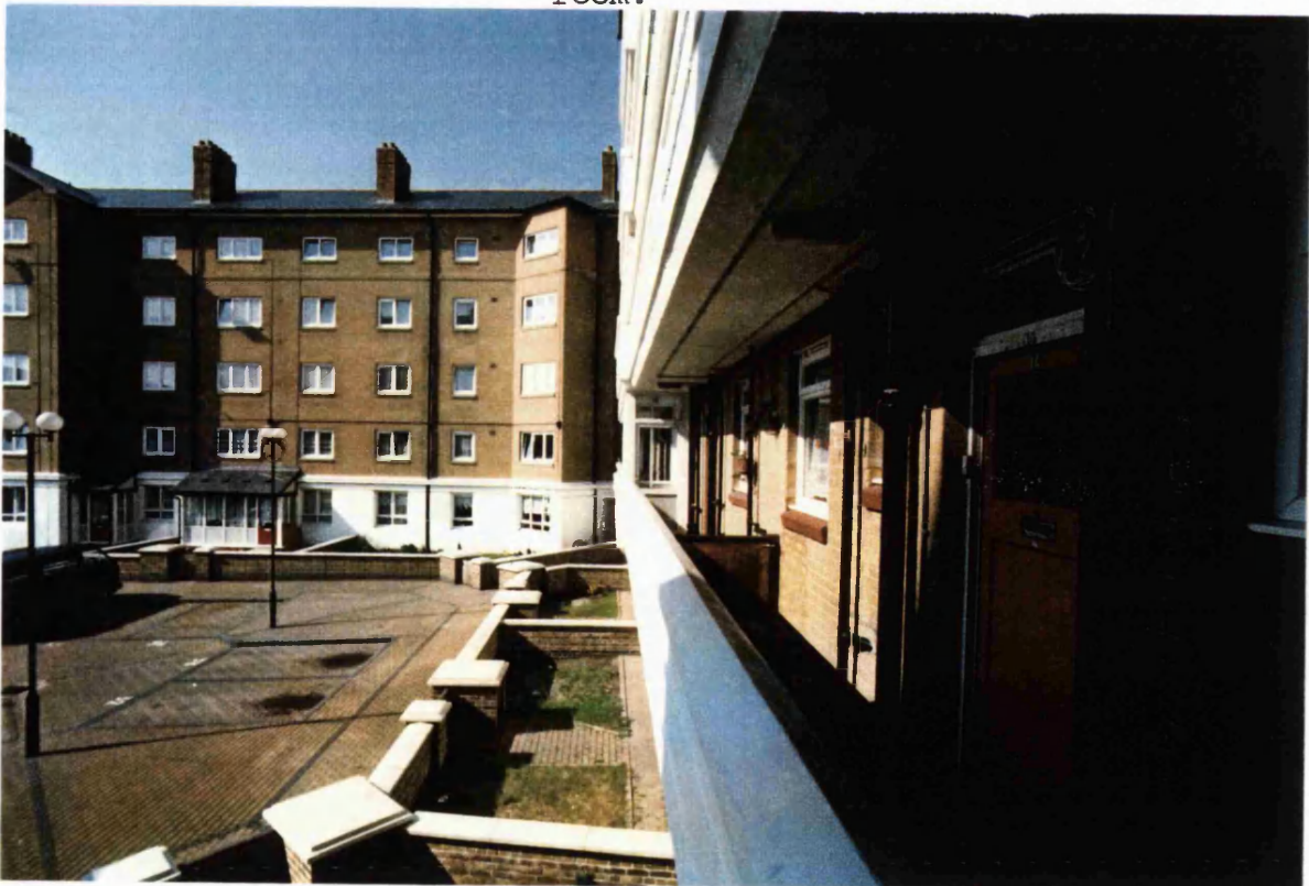
Plate 44: A view of a balcony at present and an extended room.
