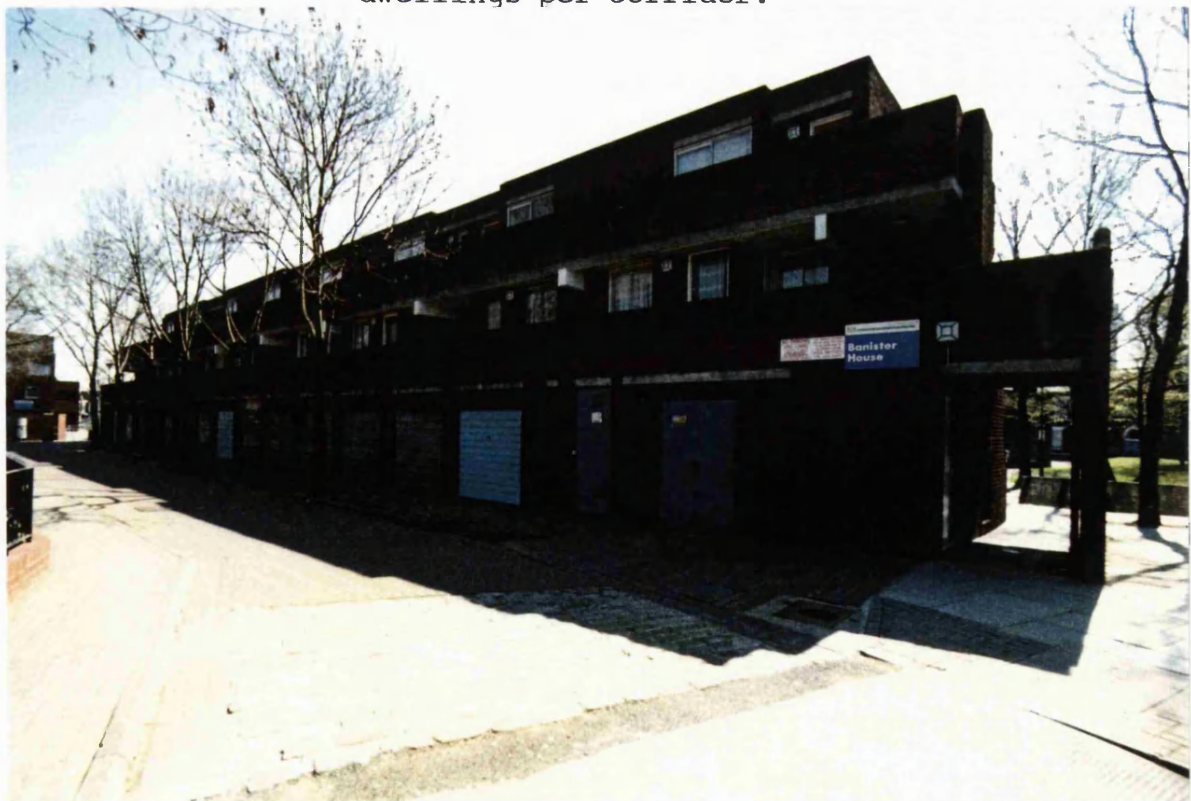
Plate 37: Bannister House which is a smaller detached blocks is located at the end of Parry Road but has not been modified as yet.
