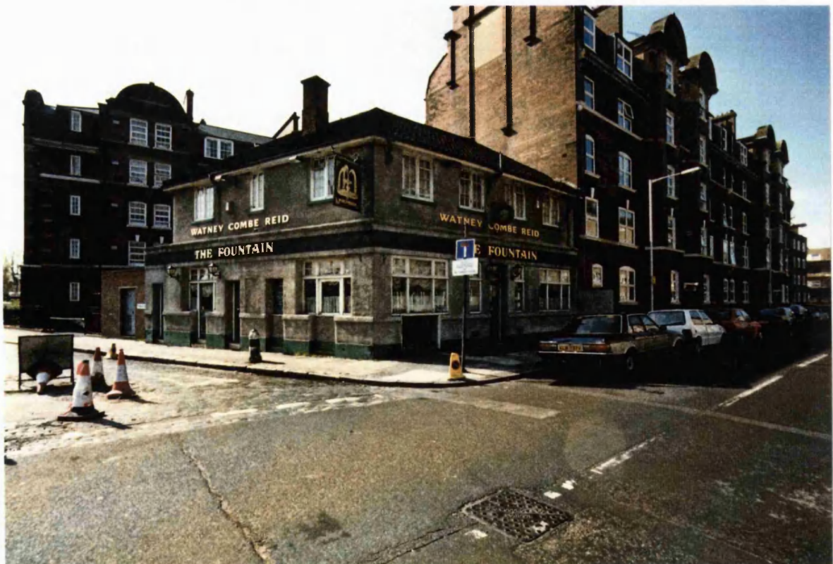
Plate 58: The Fountain Public House opposite the north block next to the neighbouring estate.
