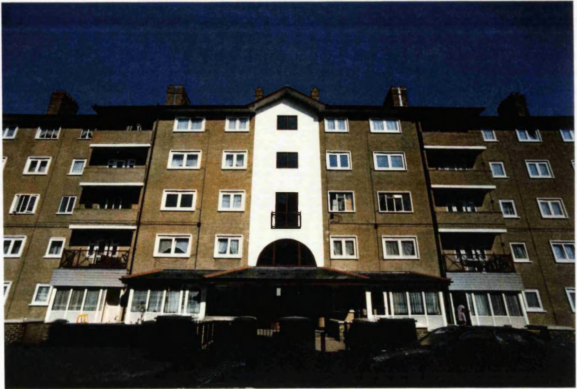
Plate 57: The front of the block on Sceptre Road where the main entrance was situated previously.
