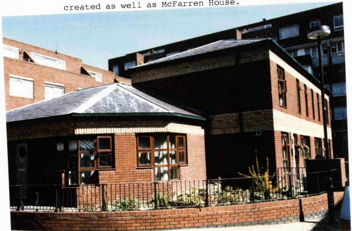
Plate 30: A new row of houses that have been created along Parry Road.
