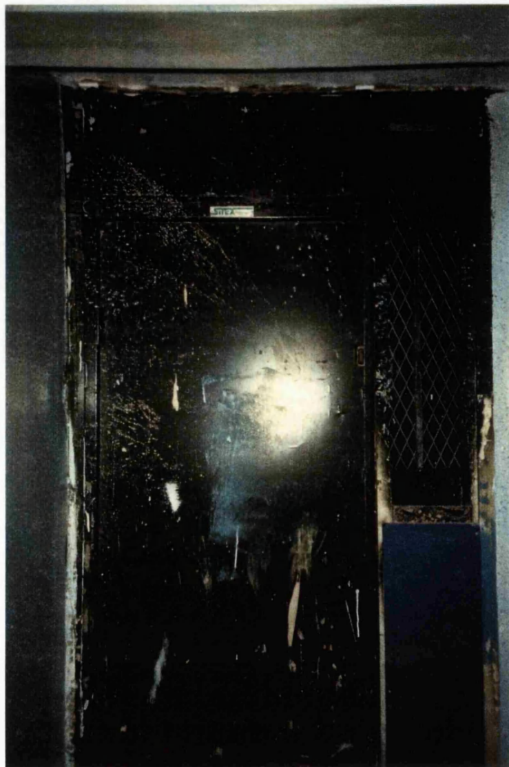
Plate 39: The door from the inside; the whole corridor was blackened in the blaze.
