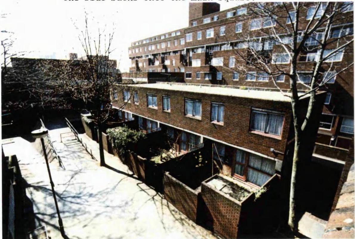
Plate 8: Redford House is a block of houses but its entrances face away from the path.
